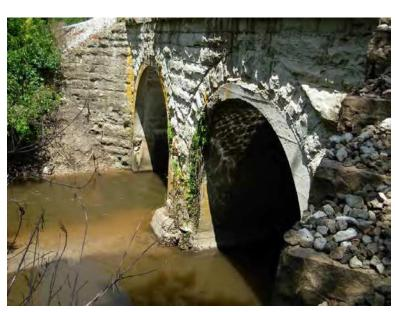
$5. \ Looking \ west \ at the \ double \ arched \ culverts \ open \ bottom \ culverts \ within \ the \ IAIS \ rail \ embankment$
