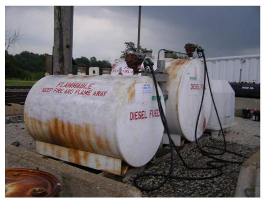
Photograph 3: Above ground storage tanks on site.
