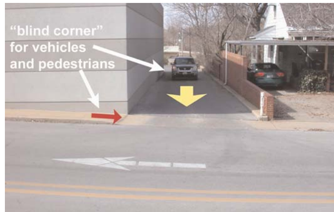
Exhibit 5-11. Driveway with very limited sight distance.
