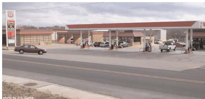
Exhibit 5-17. Undesirable wide-open driveway.
