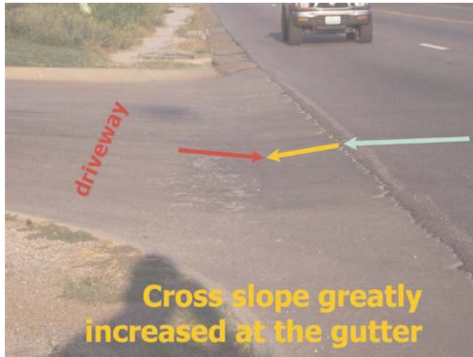
Exhibit 5-73. Increased gutter cross slope.
