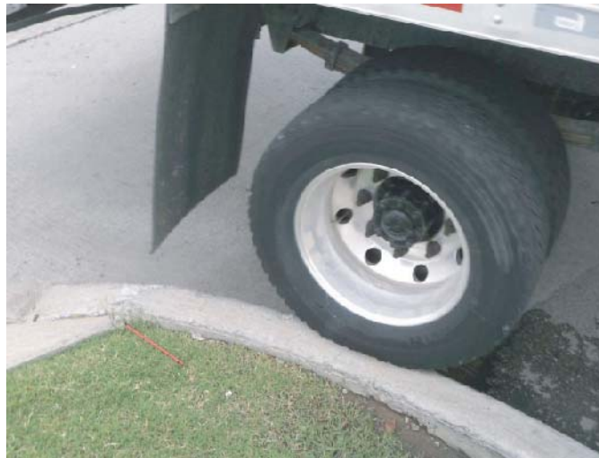
Exhibit 5-15. Effects of inadequate driveway radii.
