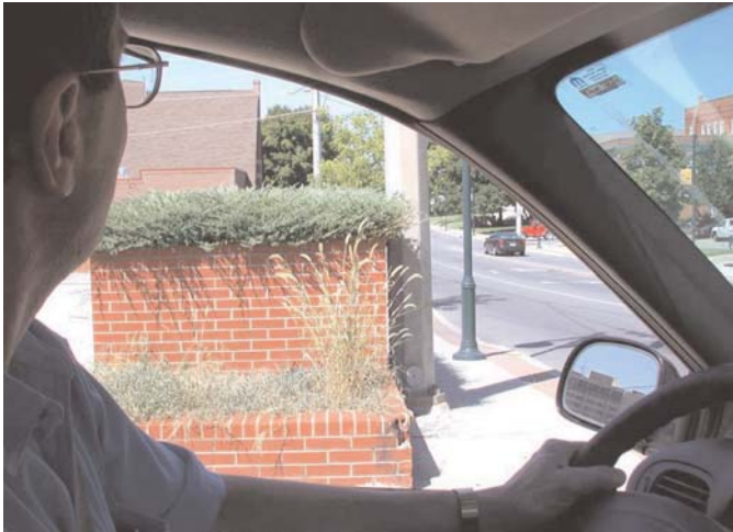
Exhibit 5-4. Placement of planter and utility pole limit the sight distance for a driveway exit.
