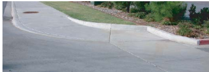
Exhibit 5-10. Unacceptable vertical curb where sidewalk crosses driveway.
