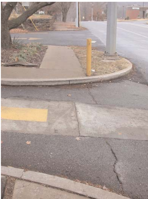
Exhibit 5-10. Unacceptable vertical curb where sidewalk crosses driveway.
