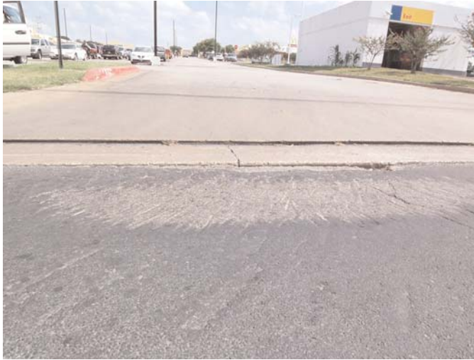
Exhibit 5-66. Driveway with multiple scrapes from underside dragging.
