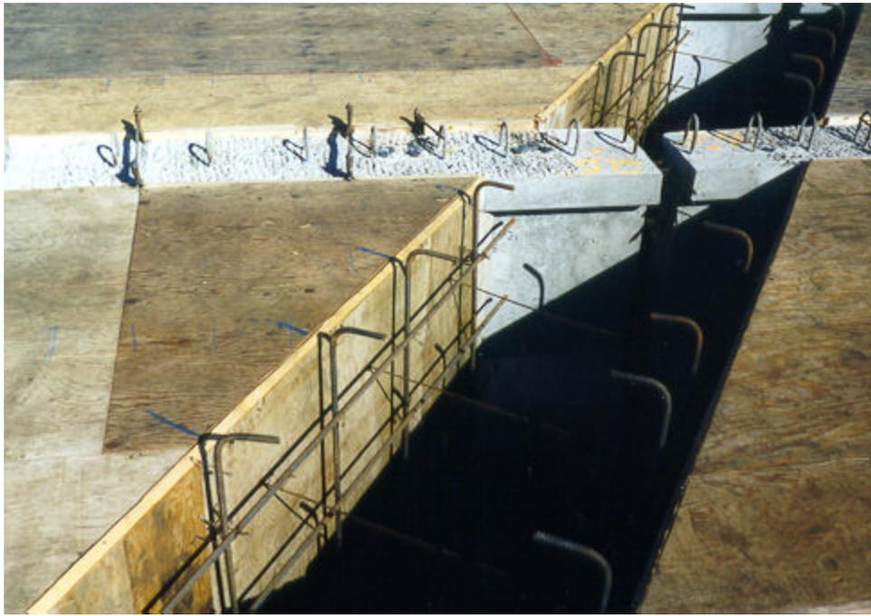
Hoop bars in pier diaphragm are properly and adequately supported.
