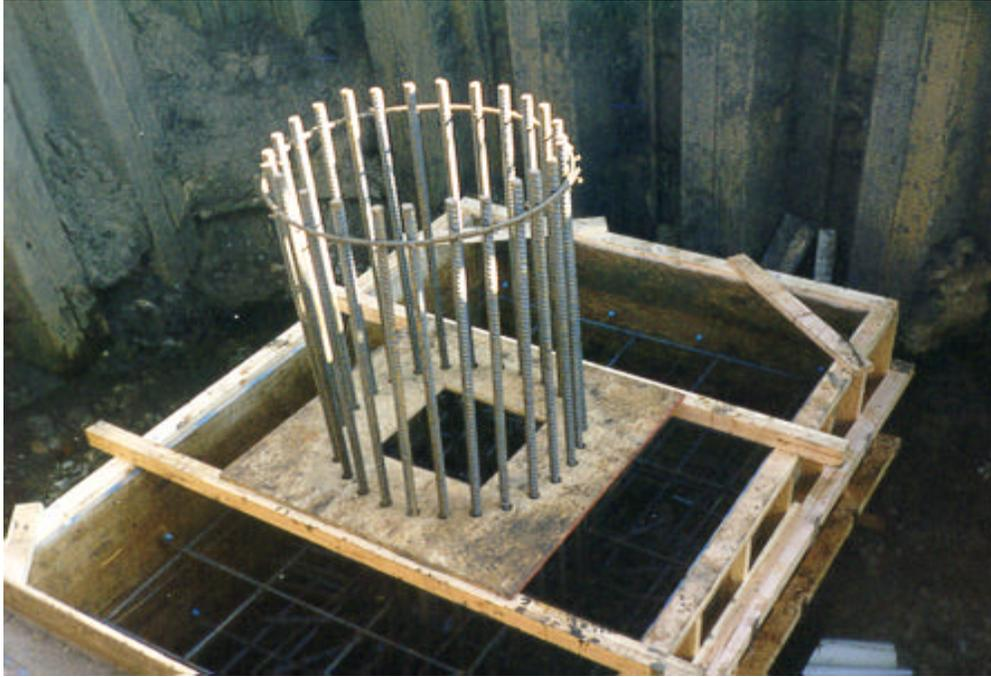
Template used in a pier footing to assure proper spacing & alignment of column steel.
