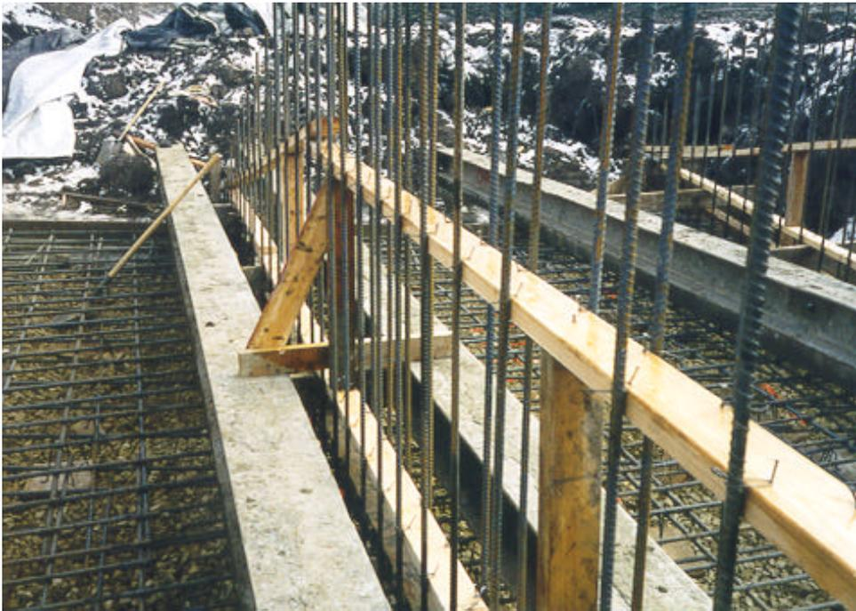
Vertical bars in a culvert wall are properly and adequately supported.
