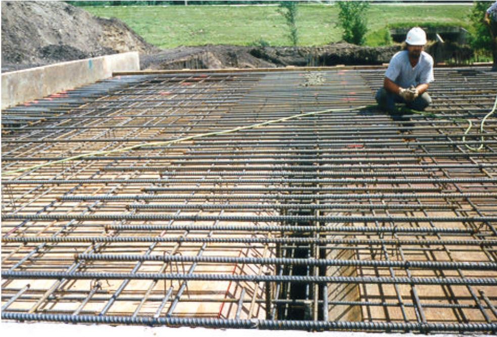
Two separate mats of reinforcing steel are independently supported in this slab for the RCB.
