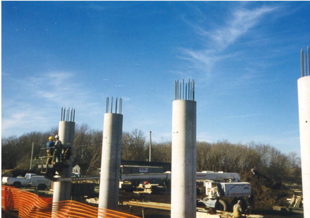
Proper spacing of vertical column bars.
