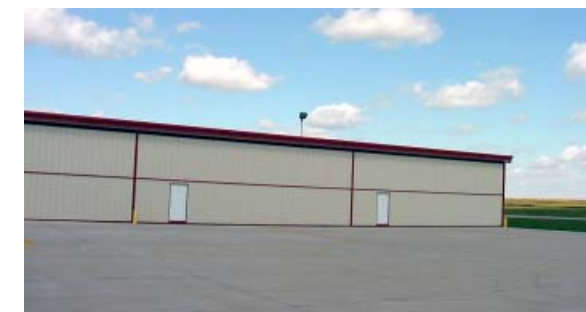
Hangars should be closed and locked.
