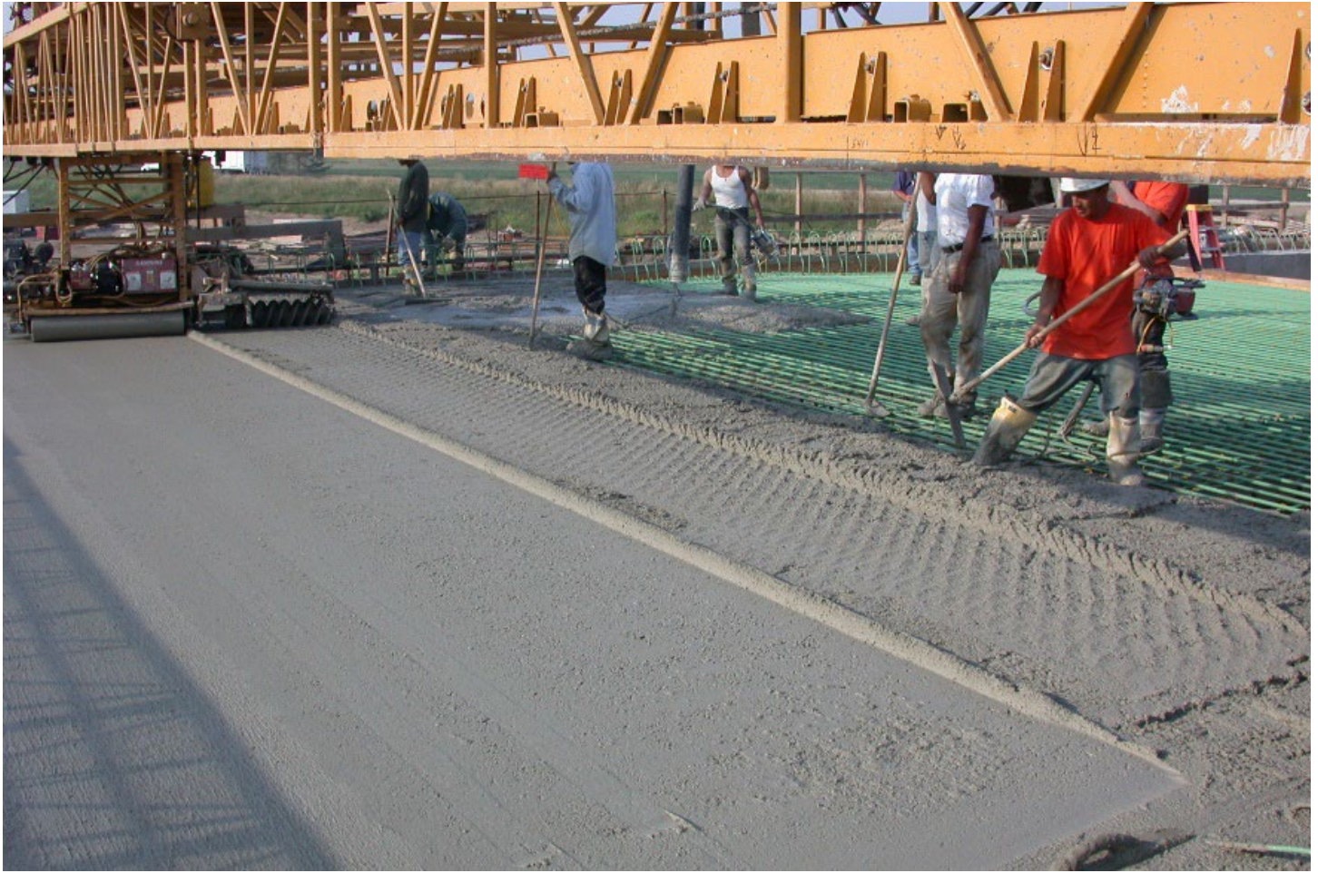
Bridge Deck Placement (Superstructure)
