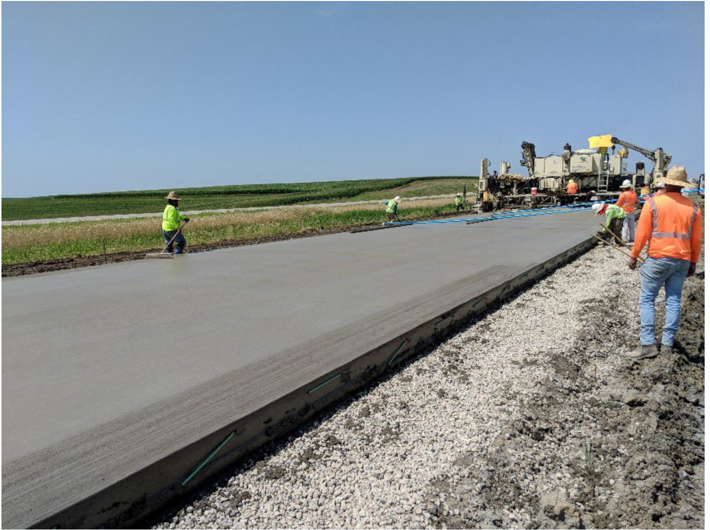
Slipform Paving
