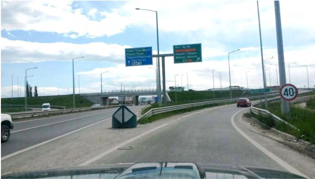
*In the picture above, the “turned-down” end treatments used for the guardrails on both sides of this ramp would not be an approved system for new installations in America. Crash tests done with similar systems here have shown that vehicles can vault up and over the “turned down” end treatment resulting in a severe crash. We are not familiar with European guardrail requirements/standards so reviewing standards may be part of your evaluation.*
