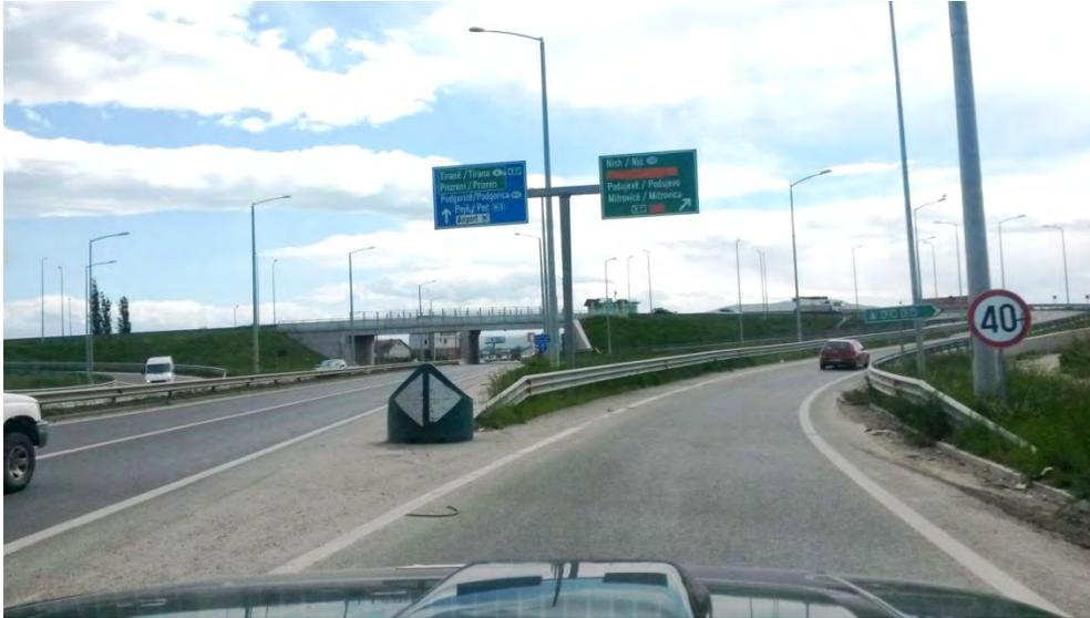
*Consider adding chevron signs behind guardrail on tight ramps.*
