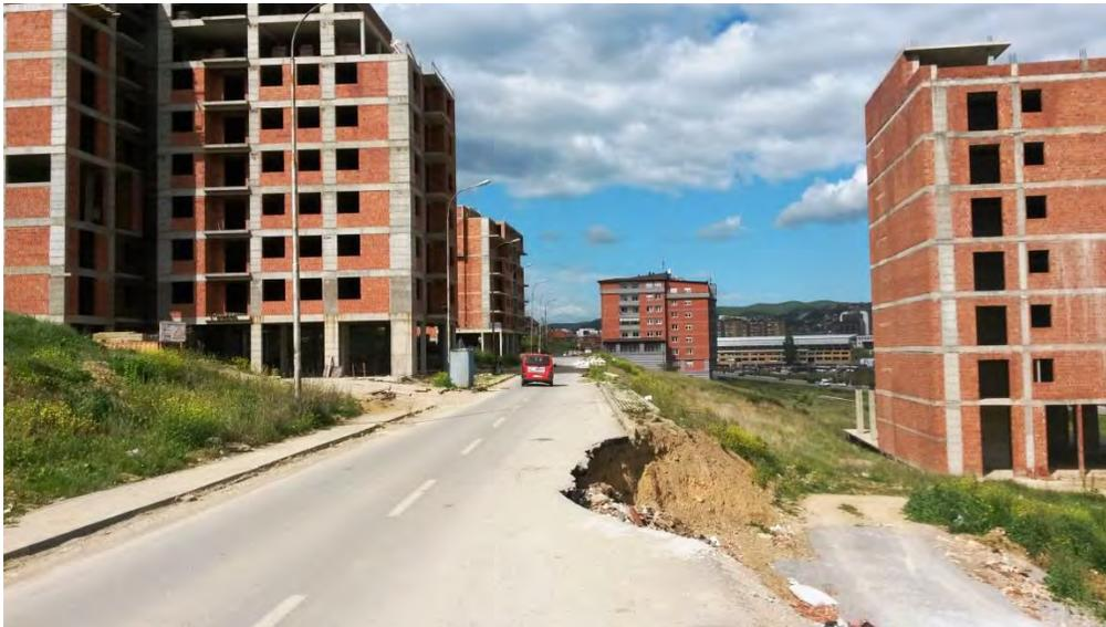
*Poor engineering design of a roadway and Illegal buildings (warning signs and traffic barriers should be placed to warn and protect roadway users of the unexpected pavement sink holes along this section).*
