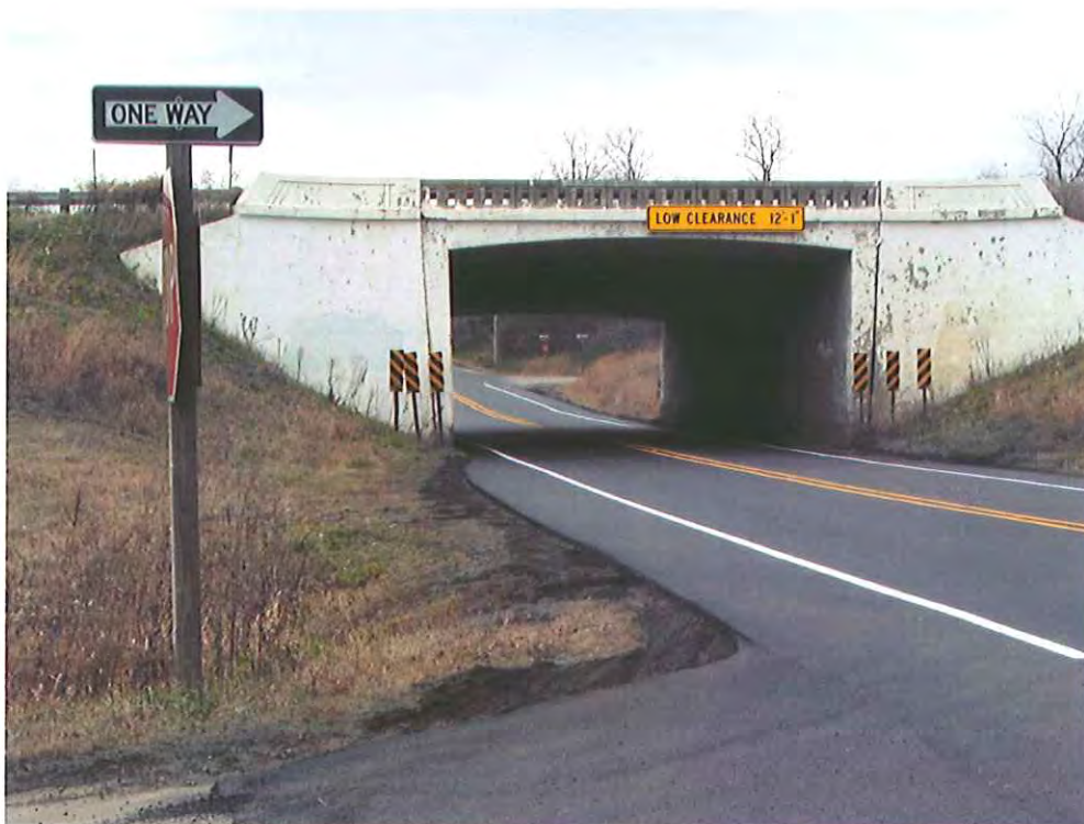
Figure 5 Limited Sight Distance from Hwy 415 SB off-ramp; Looking east from Stop Bar, middle of Ramp.
