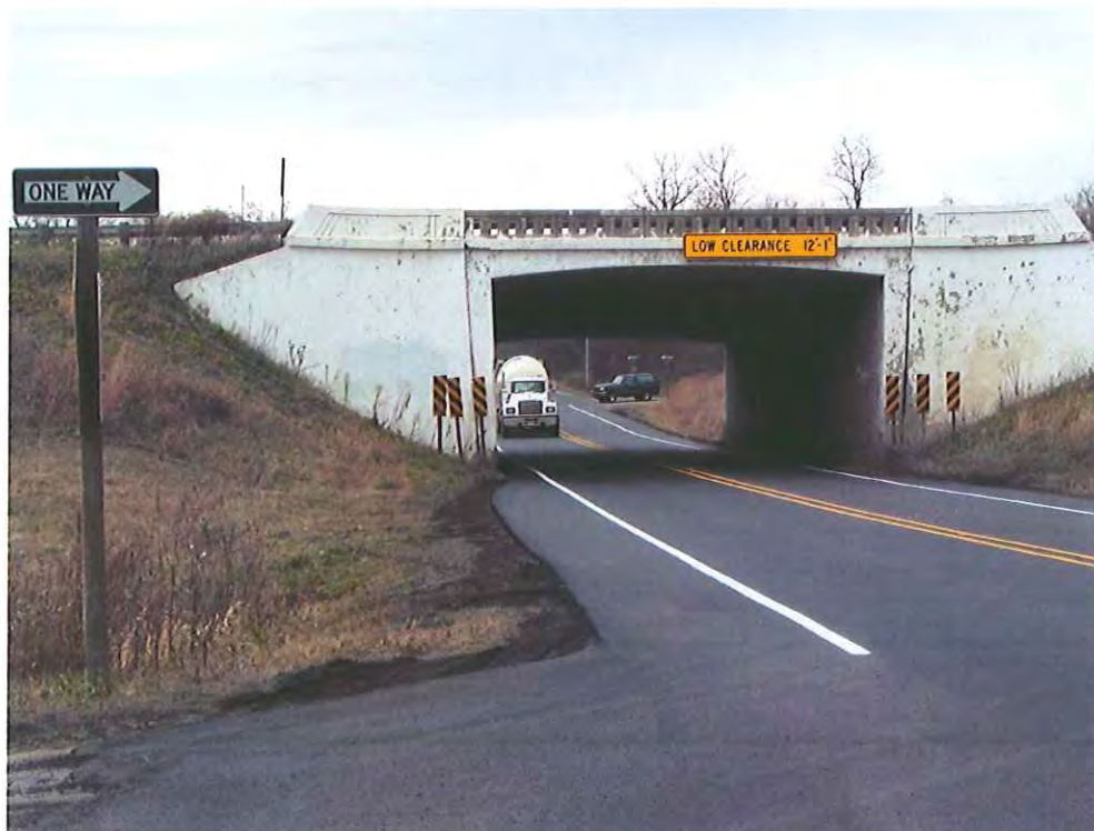
Figure 6 Limited Sight Distance from Hwy 415 SB off-ramp; Looking east from just past Stop Bar, west side of Ramp.
