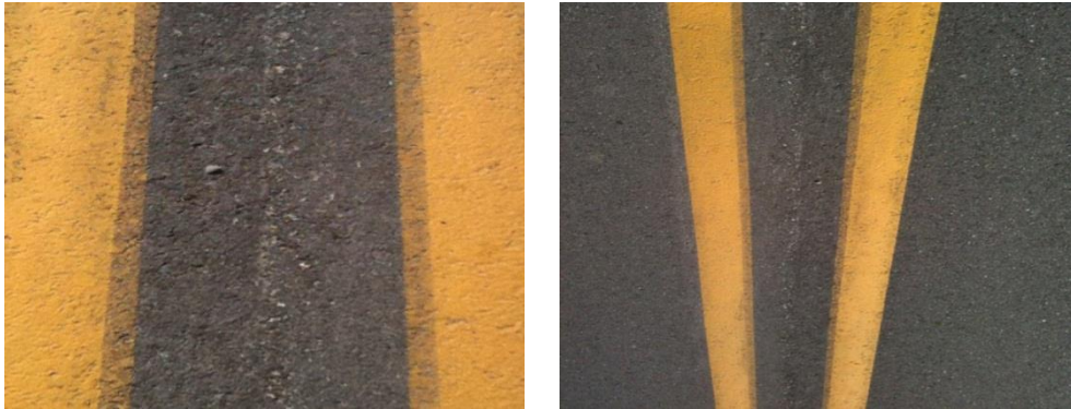
Figure 43. Longitudinal joint performance for the US 6 project
