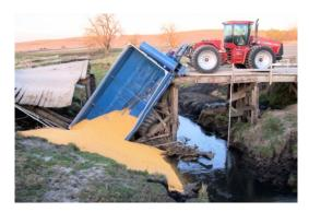
Figure 3.14. Bridge failure under grain cart (photo courtesy of Audubon County)
