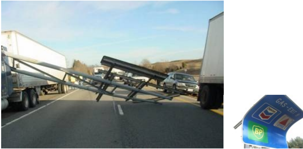
Figure 1: Damage to two highway structures due to high winds
