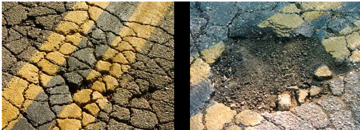
Figure 2. Alligator cracks and pothole formation
