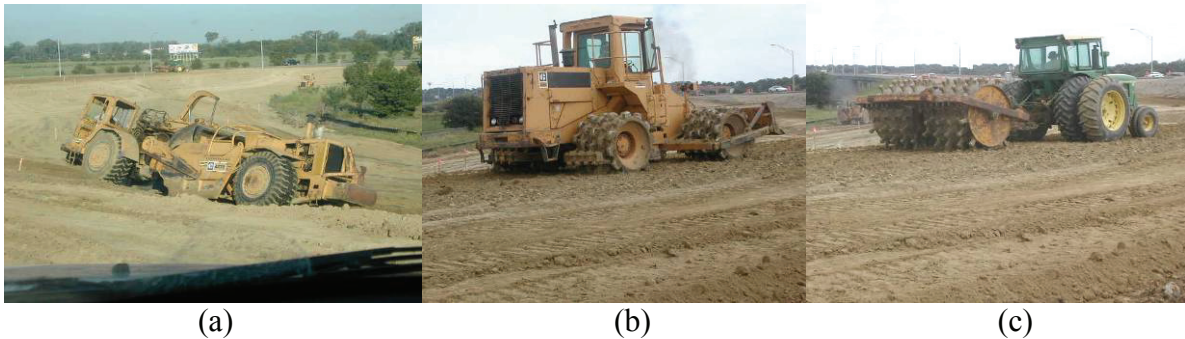
Figure 27. Equipment used on the project: (a) scraper, (b) compactor, (c) tractor-pulled roller
