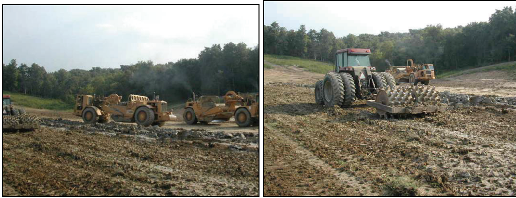
Figure 25. Scraper hauling soil and tractor-pulled sheepsfoot roller
