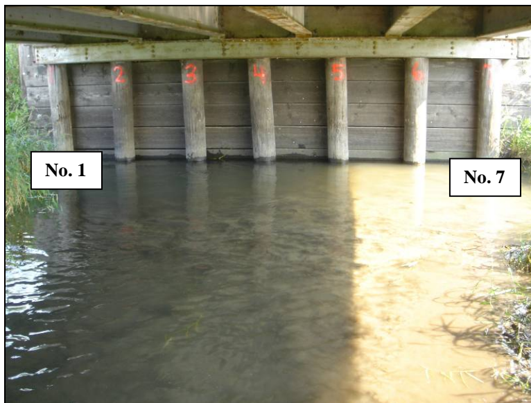
Figure 7.3. Piles denoted by numbers 1 through 7 at the north abutment (Bridge No. 7710 Boone County – July 1 2005)
