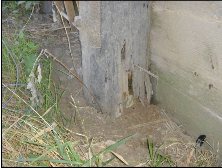
Figure 9.8. Brooming of pile No. 2 near the ground level (Bridge No. 237350 Mahaska County – October 25 2005)
