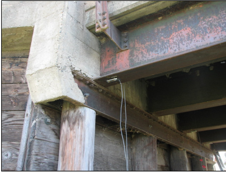
Figure 9.13. Pile cap partially resting on the timber backwall (Bridge No. 237350 Mahaska County – October 28 2005)
