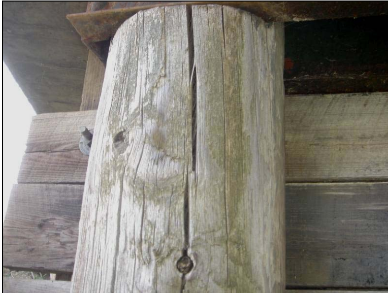
Figure 4.2. Pile cracking near the pile top (Bridge No. 1045 Black Hawk County – April 2 2005)
