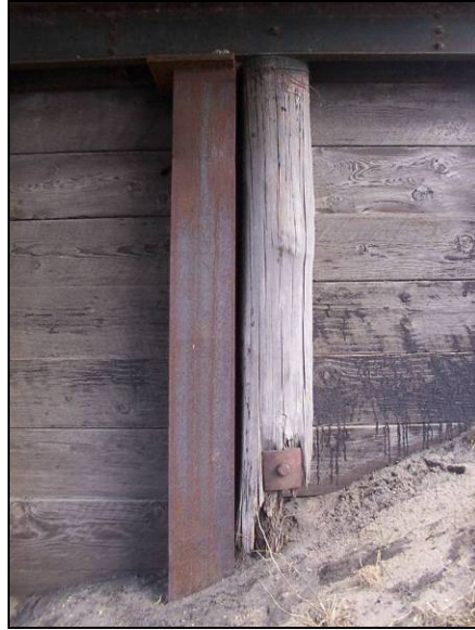
Figure 4.10. New steel pile driven adjacent to defective pile (Bridge on Indian Creek Road Black Hawk County – April 2 2005)
