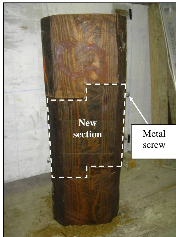
Figure 13.6. Pile section repaired using a mechanical splicing techniques
