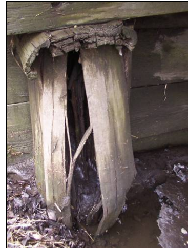
(b) Complete deterioration of pile section (Bridge No. 27-42-00 Buchanan County – February 16 2005)
