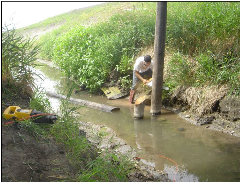
Figure 12.4. Cutting the timber piles supporting the bridge pier (Bridge No. 029070 Humboldt County – July 10 2006)
