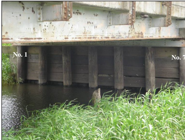
Figure 7.2. Seven supporting timber piles at each abutment with a timber backwall and double c-channel cap (Bridge No. 7710 Boone County – June 1 2005)
