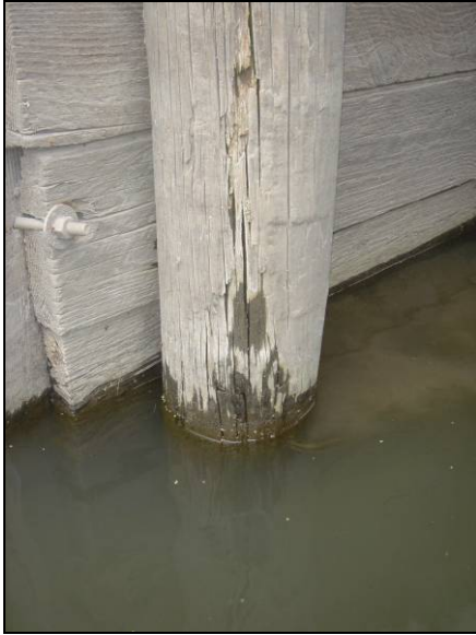
(a) Biological deterioration near the water level
