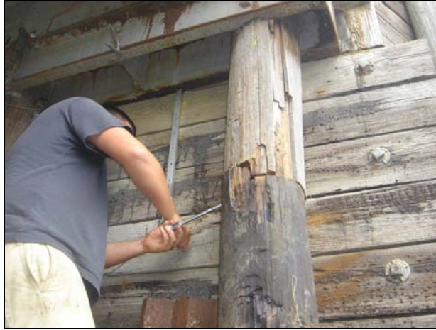
Figure 12.22. Metal screws used to connect the new section to the existing timber pile (Bridge No. 029070 Humboldt County – July 12 2006)
