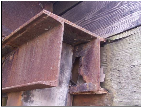
(a) Corroded steel (Bridge No. 1045 Black Hawk County – April 2 2005)
