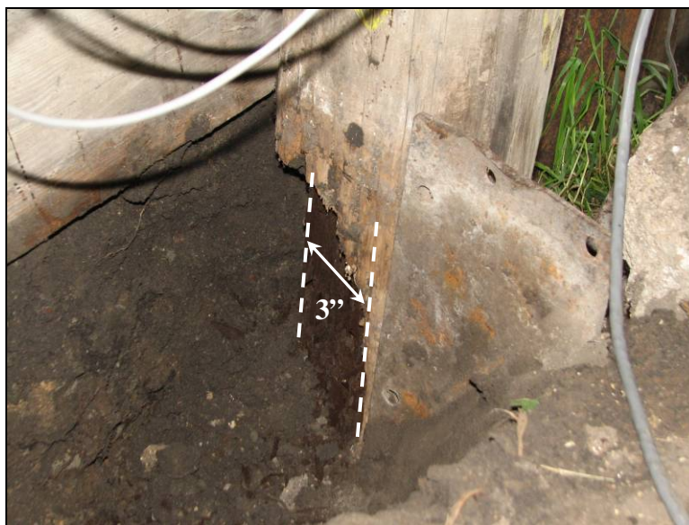
Figure 12.9. Advanced section loss at pile No. 6 at the east abutment (Bridge No. 029070 Humboldt County – July 12 2006)
