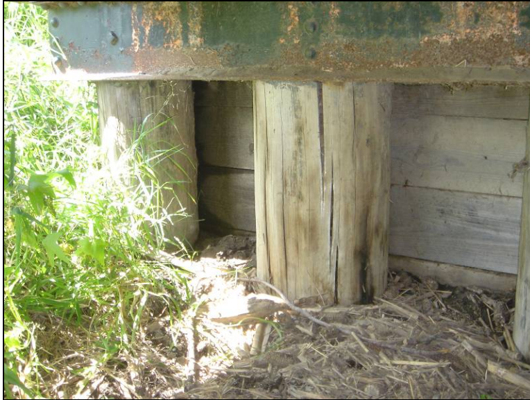
Figure 8.6. Hammer sounding and probing revealed a hollow core at pile no. 2 at the north abutment (Bridge No. 243470 Marshall County – June 22 2005)
