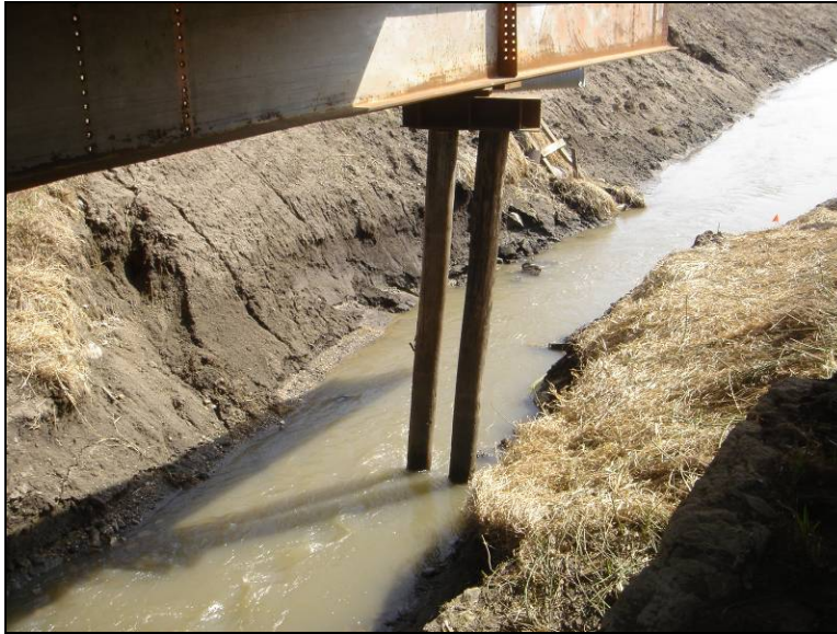
Figure 12.3. Center pier supported by 2 timber piles on each side of the bridge (Bridge No. 029070 Humboldt County – April 4 2006)
