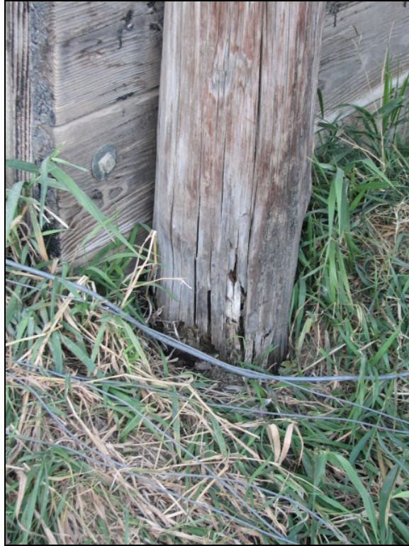
Figure 9.4. Biological deterioration of pile No. 1 at the ground level (Bridge No. 237350 Mahaska County – October 25 2005)
