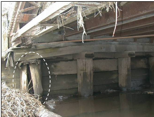
(b) Complete deterioration of pile section (Bridge No. 27-42-00 Buchanan County – February 16 2005)
