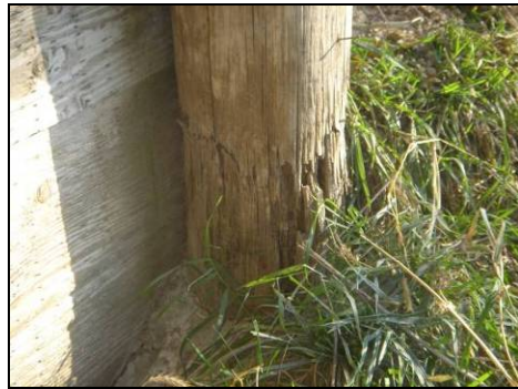
(b) Brooming of pile at the east end of the north abutment
