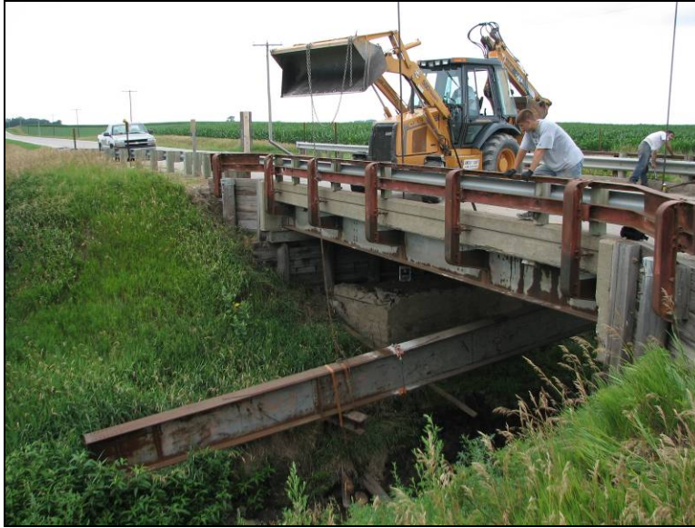
Figure 12.5. Lowering the steel girder (Bridge No. 029070 Humboldt County – July 10 2006)
