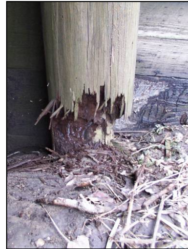
(a) Reduction of pile cross section (Bridge No. 13-42-06 Buchanan County – February 16 2005)
