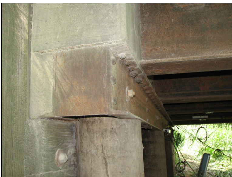
Figure 11.15. Partial bearing of the pile cap on the southeast abutment backwall (Bridge No. 237380 Mahaska County – May 27 2006)
