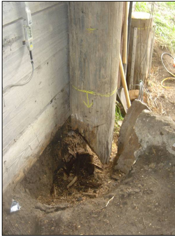
Figure 12.20. A section of Pile no. 6 removed near the ground level (Bridge No. 029070 Humboldt County – July 12 2006)
