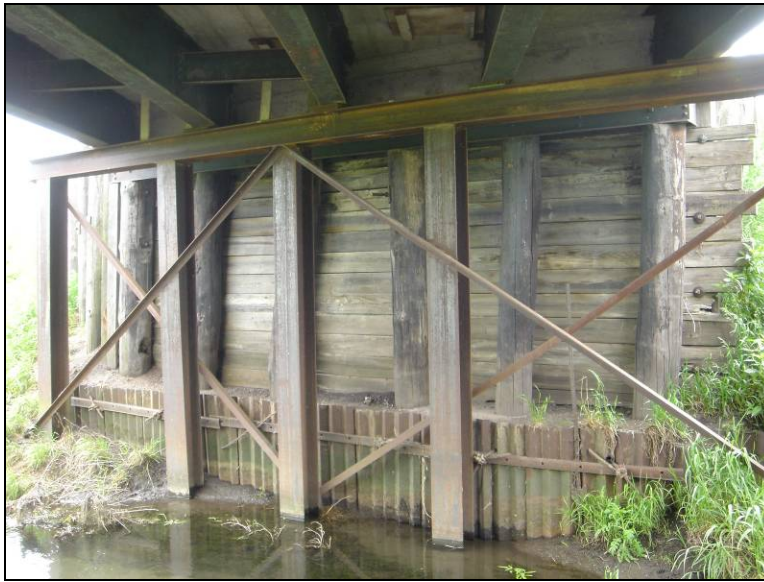
Figure 4.14. Steel piles used to replace deteriorated timber abutment (Bridge in Boone County – June 1 2005)
