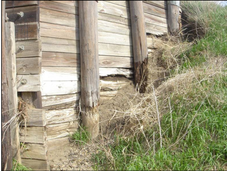
Figure 10.4. Severe deterioration observed at the northeast wingwall piles (Bridge No. 094680 Carroll County – April 15 2006)
