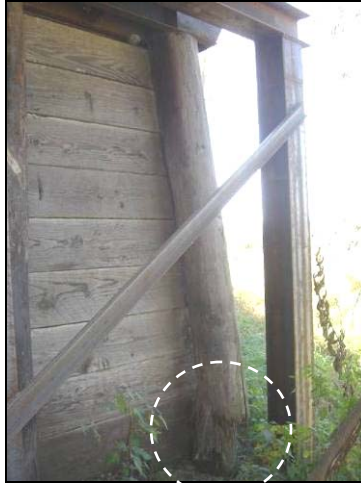
(a) Separation of pile section (Bridge No. 23-70-00 Mahaska County – July 8 2005)
