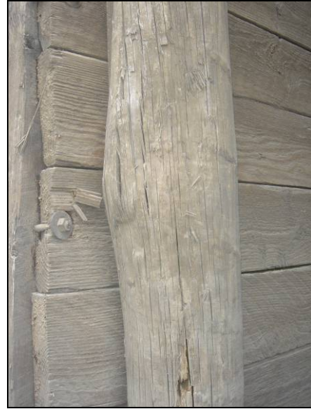
(b) Bulging of timber fibers
