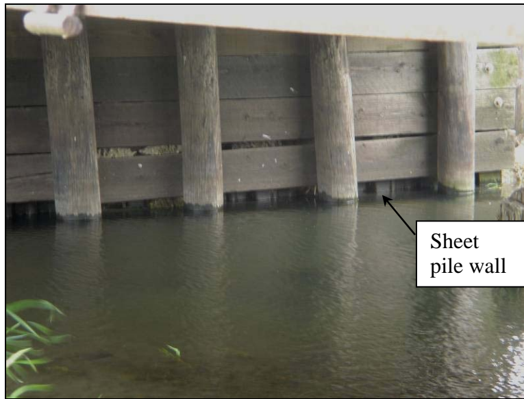
Figure 7.8. Sheet pile wall driven behind the south abutment to prevent backfill erosion (Bridge No. 7710 Boone County – June 1 2005)
