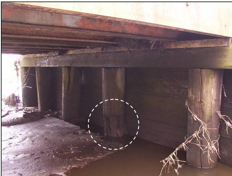
Figure 4.3. Reduction of pile cross section by abrasion from flowing debris and ice (Bridge No. 27-74-23 – February 15 2007)
