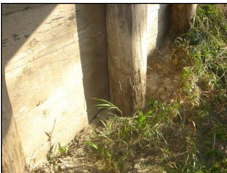
(c) Soft pile section with high moisture near the ground level
