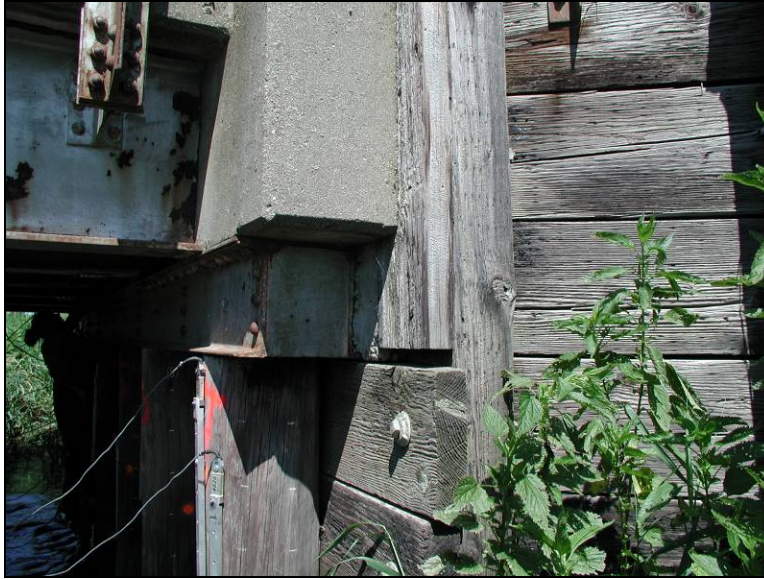
Figure 7.13. Possible eccentric loading caused by misalignment of pile cap (Bridge No. 7710 – Boone County)
