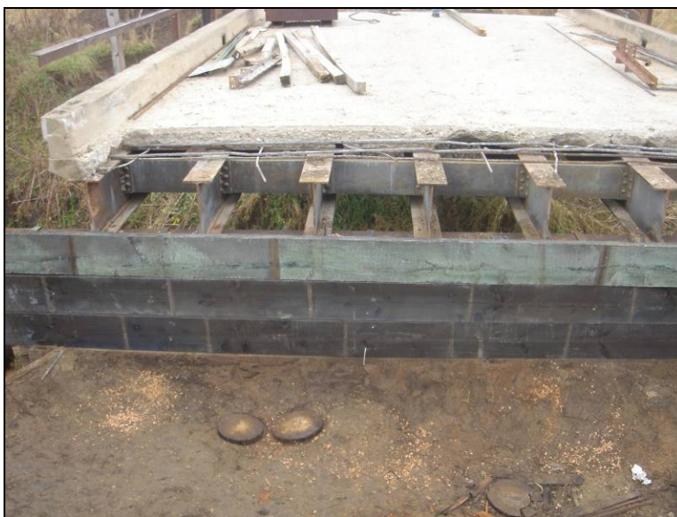
Figure 4.12. A section from the concrete deck is removed for driving timber piles (Bridge No. 31-72-50 Tama County – September 8 2005)
