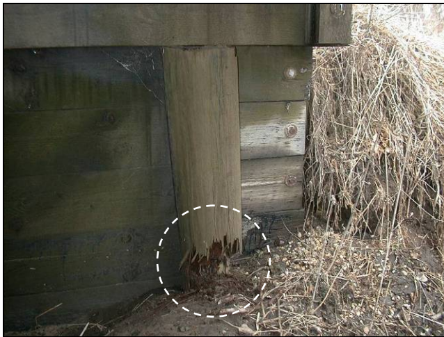
(a) Reduction of pile cross section (Bridge No. 13-42-06 Buchanan County – February 16 2005)
