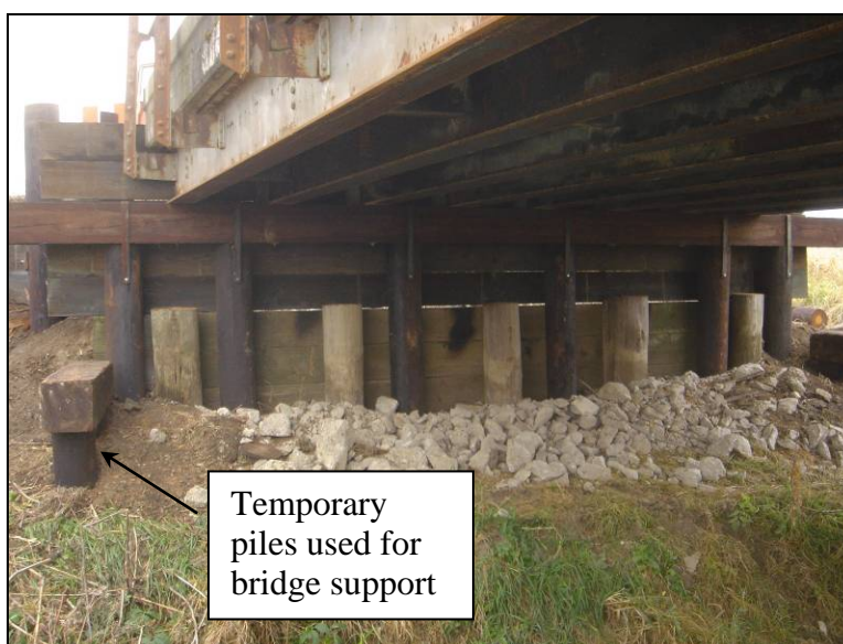
Figure 4.13. New timber abutment system constructed at the north side (Bridge No. 31-72-50 Tama County – September 8 2005)
