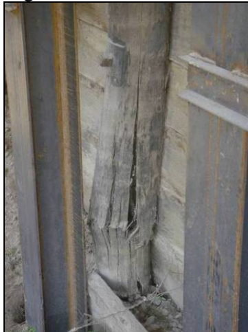
(c) “Mushrooming” of fibers at a hollow section (Bridge No. 23-70-00 Mahaska County – July 8 2005)
