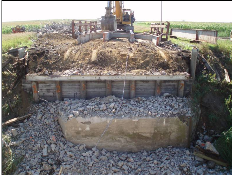
Figure 12.12. Removing the bridge super structure – looking west (Bridge No. 029070 Humboldt County – July 28 2006)
