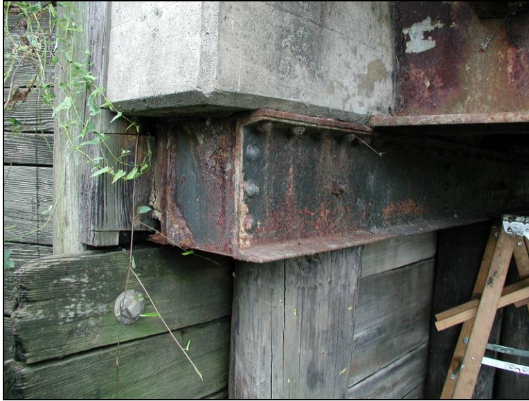
Figure 8.18. Pile cap partially resting on the timber backwall (Bridge No. 243470 – Marshall County – July 28 2005)
