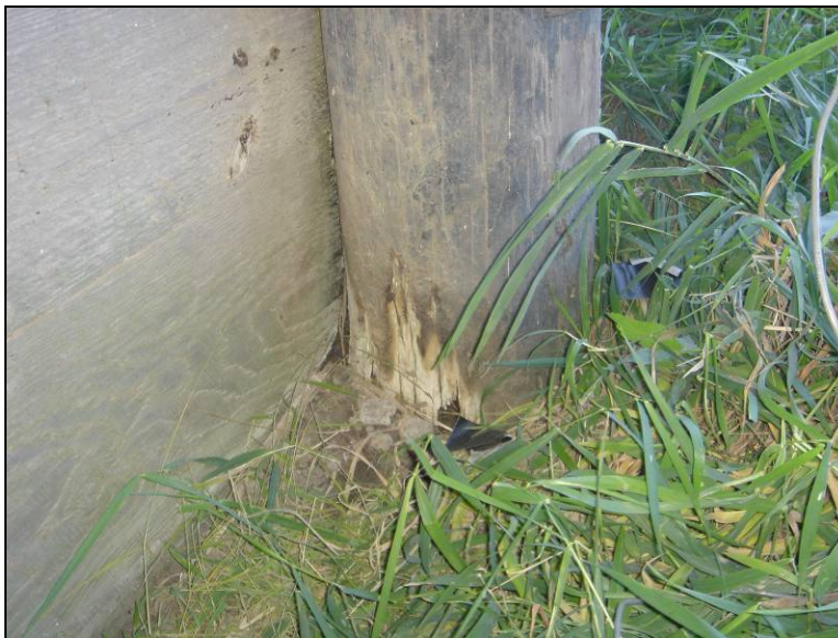
Figure 9.9. Rotting observed at pile No. 5 (Bridge No. 237350 Mahaska County – October 25 2005)
