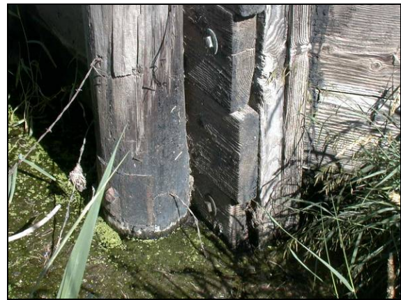
(b) Soft section near the water level
