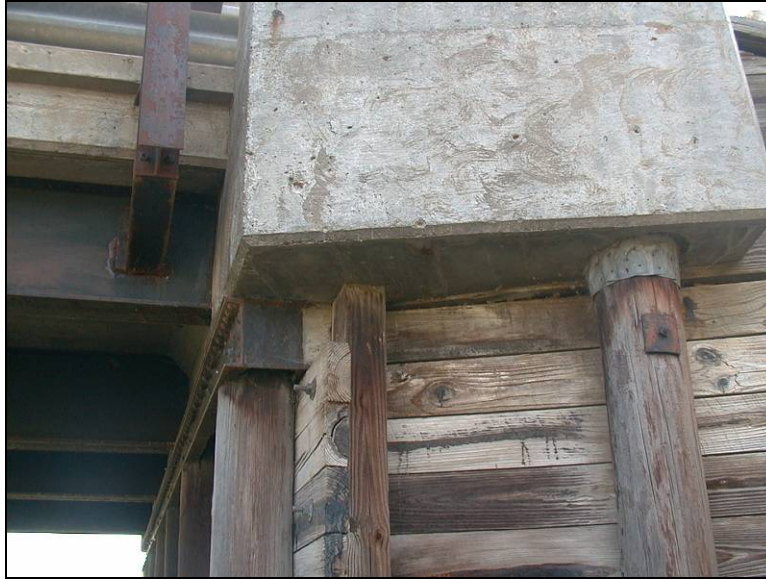
Figure 10.14. Pile cap partially resting on the backwall (Bridge No. 094680 Carroll County – May 16 2006)
