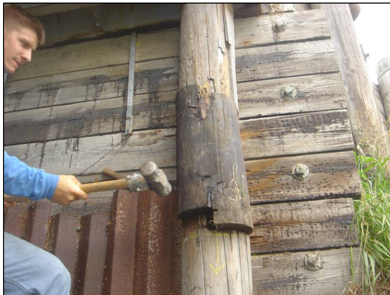
Figure 12.21. Installing a new timber section to repair pile no. 7 (Bridge No. 029070 Humboldt County – July 12 2006)
