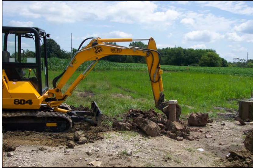
(a) Exhumation of piles with excavator
