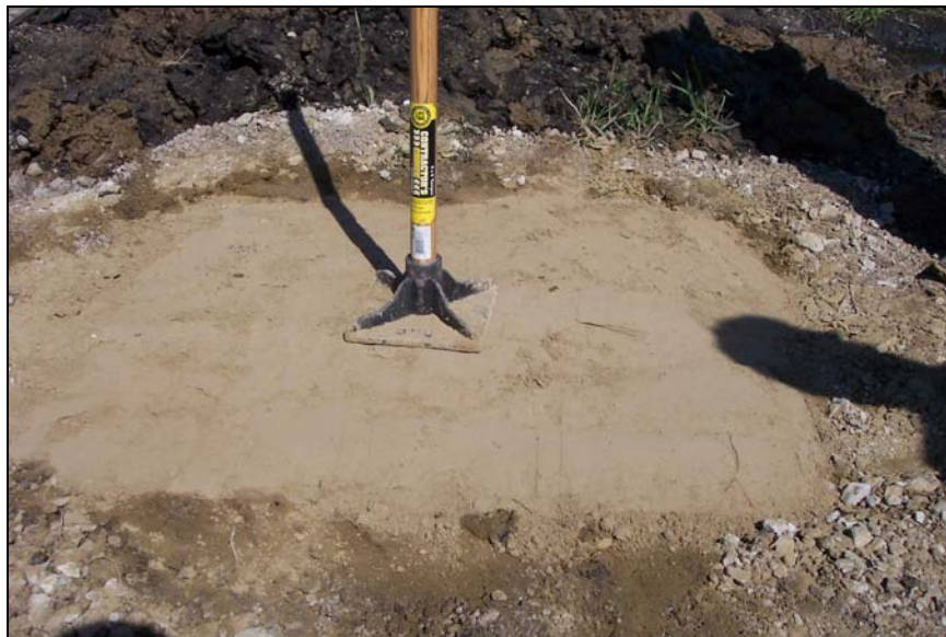
Figure 34. Compaction of soil control soil pads
