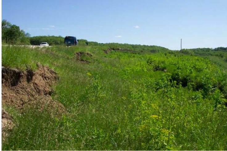
(a) Looking south, showing the scarp and graben of the slope (photo taken by Thompson, 05/26/04)
