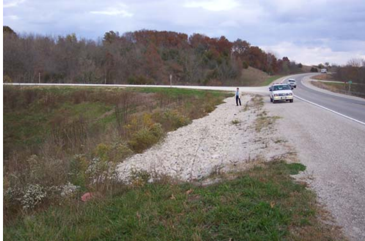
(a) Looking east, showing the rip-rap (photo taken by Thompson, 10/27/03)
