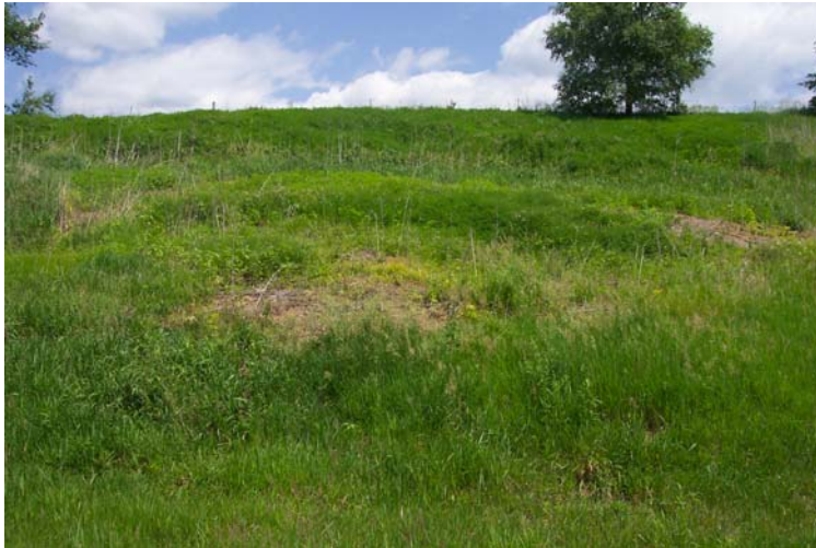
(b) Looking east, showing the bulge and scarp of the slope (photo taken by Thompson, 06/04/04)
