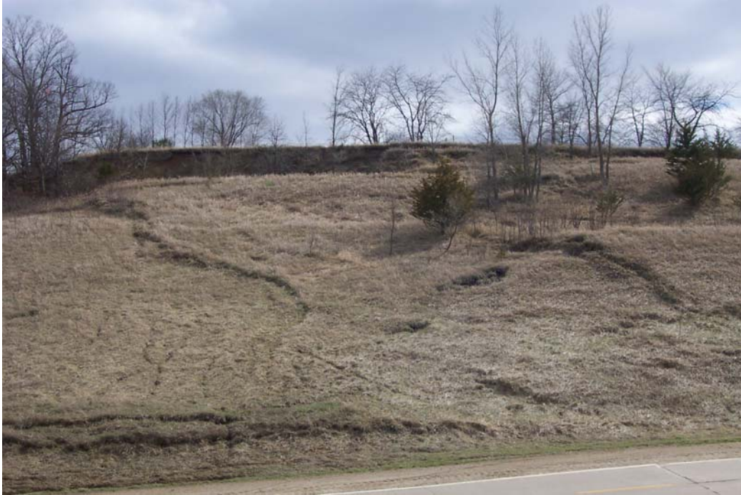
(d) Looking southwest, scarps of the slope 11 (photo taken by Thompson, 03/30/04)
