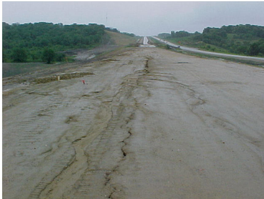
Figure 1. Existing slope failure at Highway 330 in Jasper County, Iowa (White 2003)
