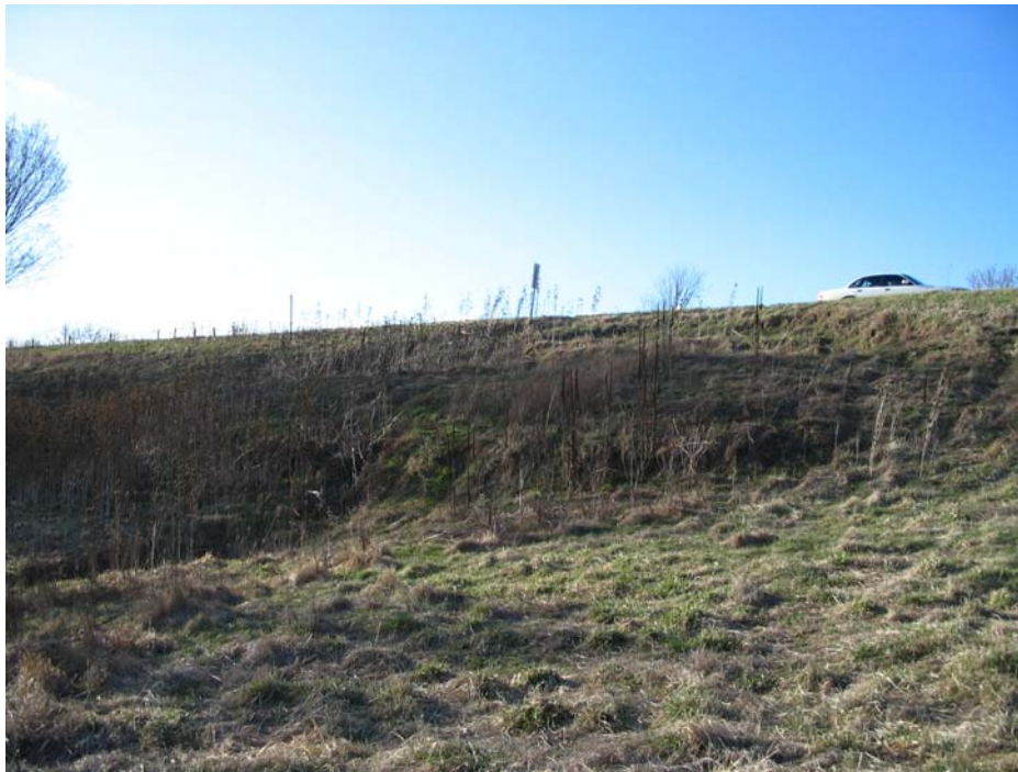
(b) Looking northwest, close view of the bulge and the scrap (photo taken by Yang, 04/01/05)
