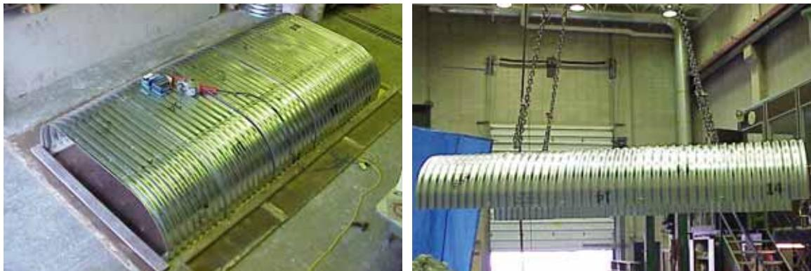
Figure 4.10. Assembly of the formwork batteries.
