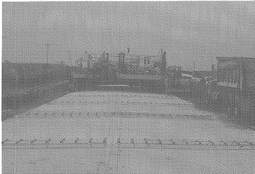
The tracks of the paver ran on the subbase when the pavement was placed
