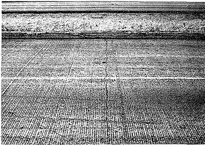
Figure 14 Reflected Transverse Crack in Resurfacing
