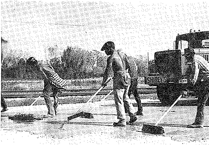
Figure 7 Workmen Spreading Grout
