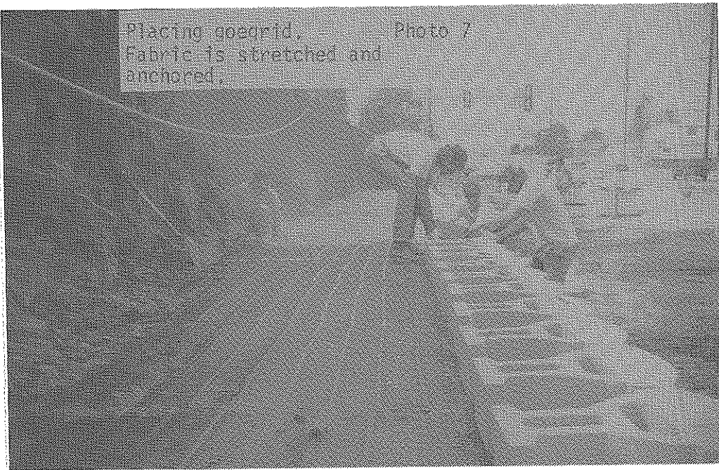
Overlap of geogrid at wall end anchorage.
