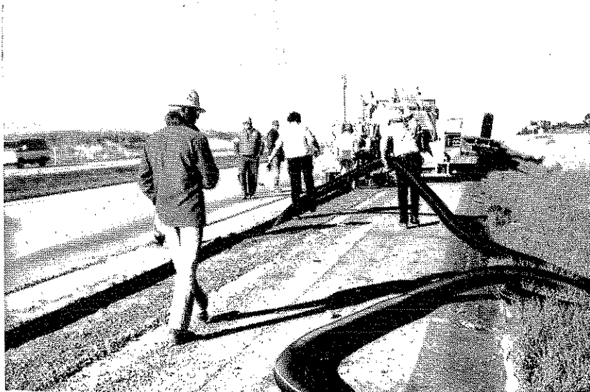
Figure 4: Hand Placement of the Tubing
