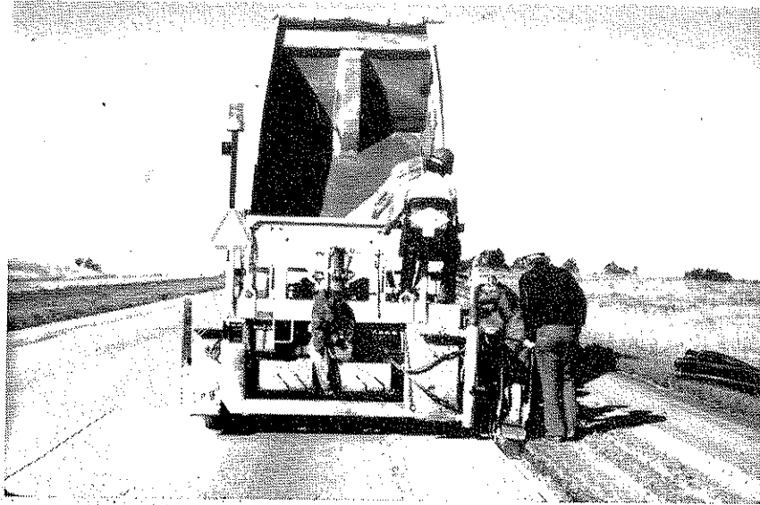
Figure 5: Blawnox RW-38 Placing Porous Backfill
