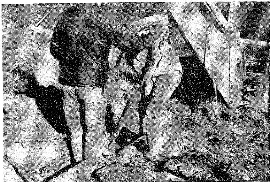
Figure 10: Tamping Earth Fill Around the RF-22 Outlets
