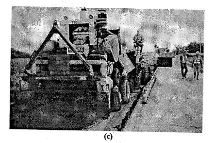
Figure 2: Operating CIR Train (Carroll County 1996 - moving right to left) (a) milling machine (b) screening unit and pugmill (c) laydown machine
