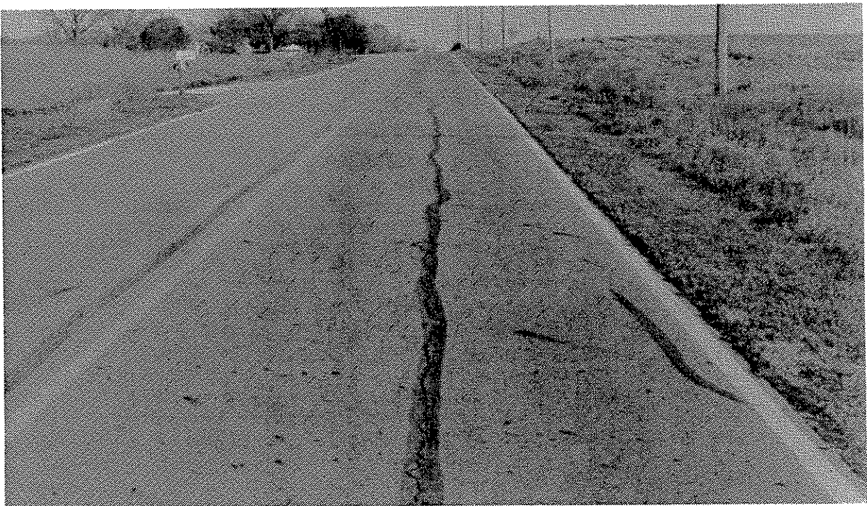
APFA Base Sections With Surface Cracks
