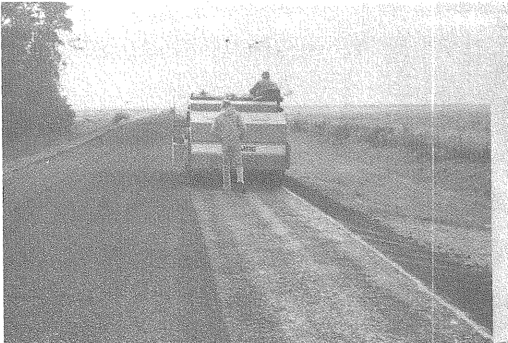
Figure 6. Compaction of road mix section
