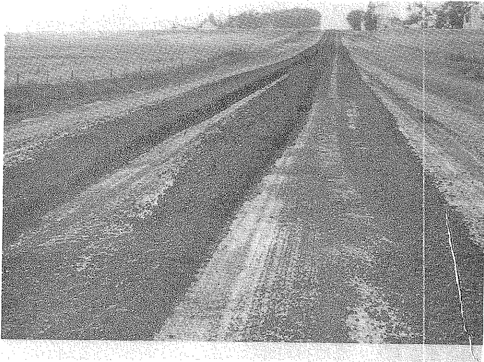
Figure 5. SC-800 road mix left to aerate after mixing.
