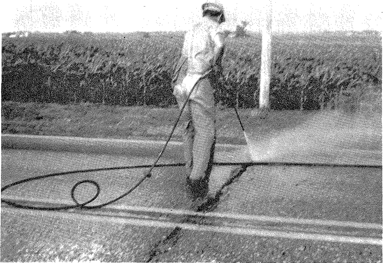
Figure 7 - Waterblast Routing of a Transverse Crack
