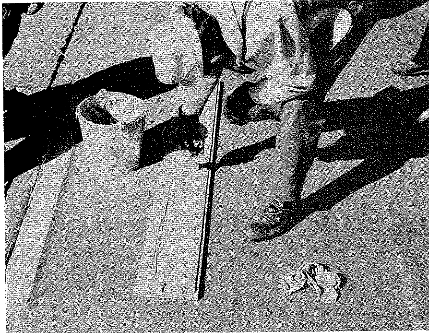
Figure 5. Application of epoxy to reflector unit and to groove in pavement
