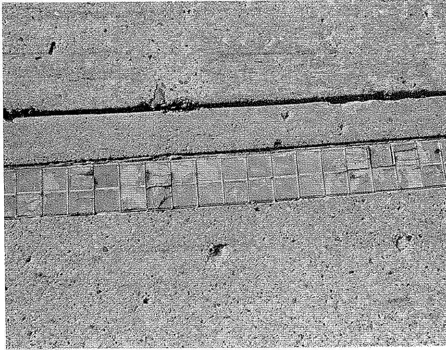
Figure 10. A reflector unit in "poor" condition
