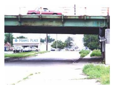
Photo 3. Bridge lacks established vertical clearance over  $10^{\rm th}$  Street
