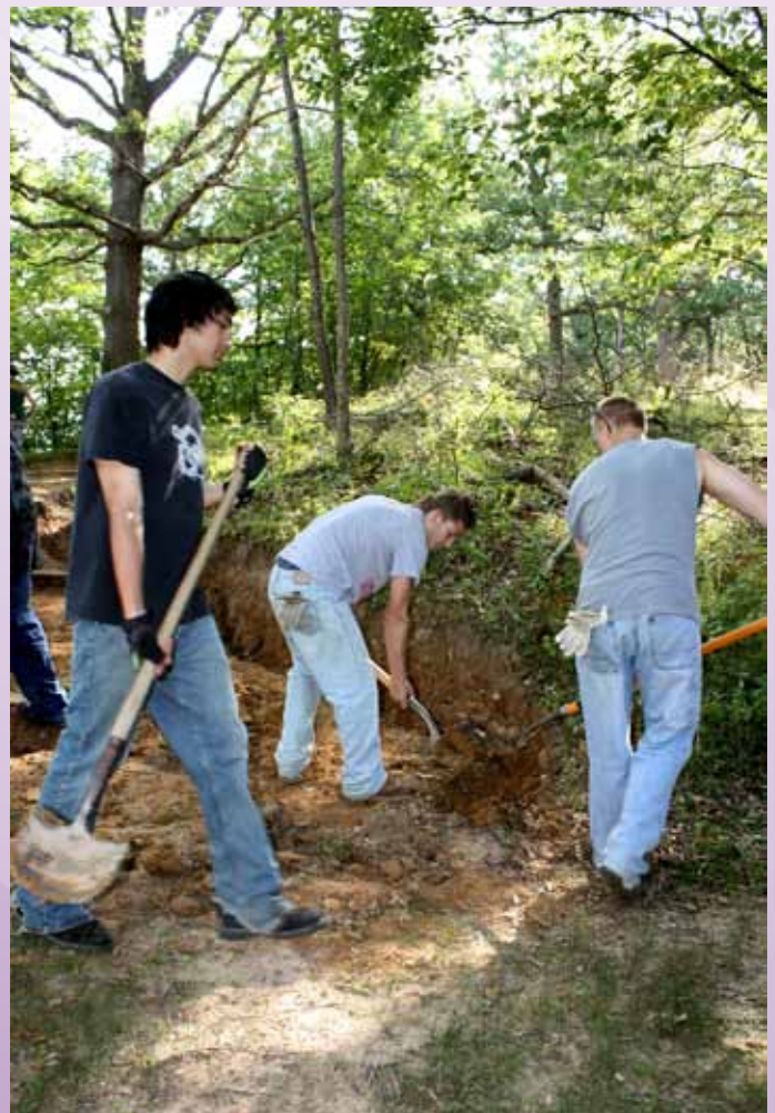
This hand-dug trench will enhance safety on the Woodpecker Trail near the Coralville Reservoir by diverting rain water that used to damage the trail surface.
