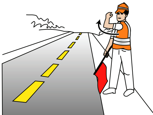
Figure 10 Using a flag to release traffic in emergencies
