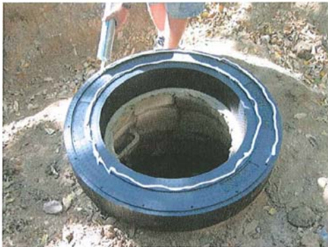
7. Apply a ¼" bead of M-1 adhesive to each of the tongues. Install the next Grade Ring if required, grooves down or proceed to step 8.
