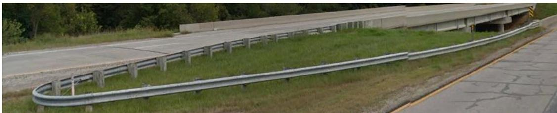
As noted above, new and existing guardrail should not be combined. If any part of an installation needs to be replaced, replace the entire installation.
