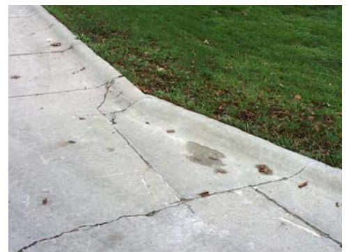
Jointing for tie-ins must be carefully considered
