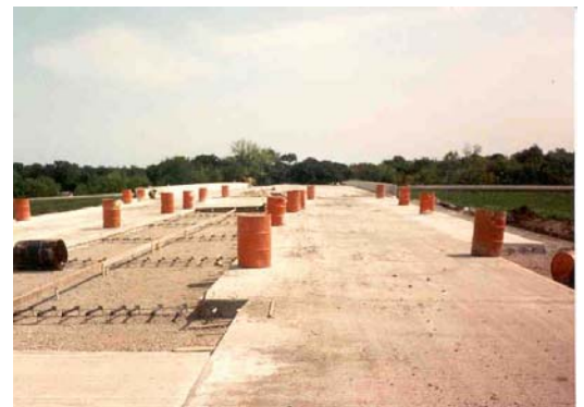
Box outs in multilane paving
