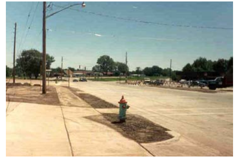
Fire hydrant placed too high
