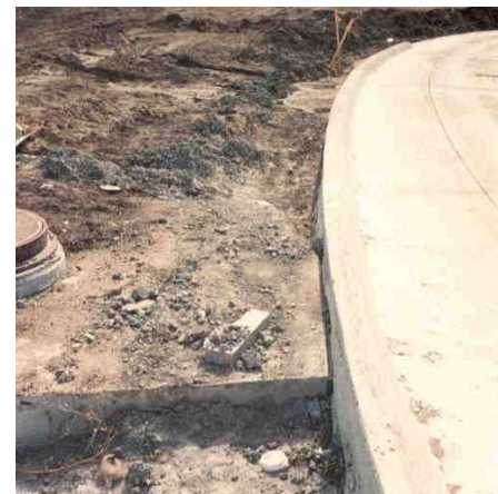
Pavement edge next to a utility access
