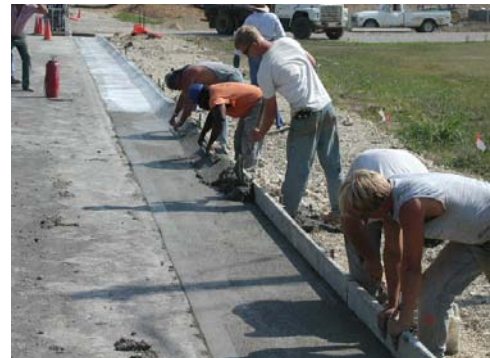
Hand placement of the curb
