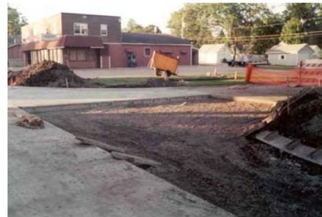
Radii are irregular shapes and normally are constructed using hand pours
