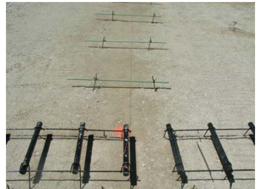
Placement of tie bars and CD baskets prior to paving
