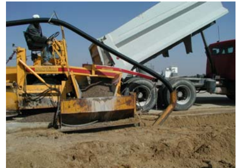
Mule placing the subdrain and porous backfill
