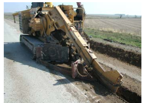
Excavation of the subdrain trench
