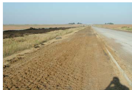
Shoulder after compaction and prior to final finishing
