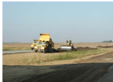
Depositing and spreading earth shoulder material
