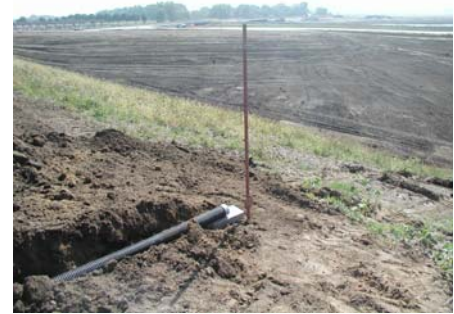
Outlet is marked by a metal post
