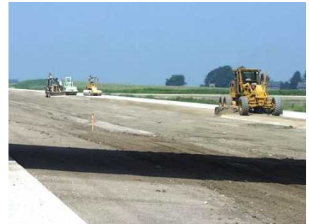
Final shoulder finish with compaction and brooming of slab
