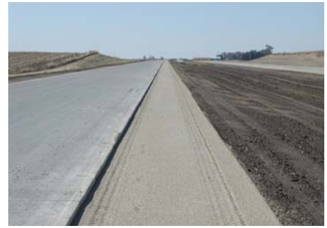
Granular shoulder ready for the final lift
