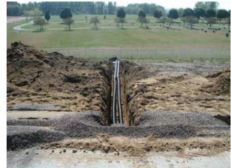
Outlet placed out to the toe of the foreslope
