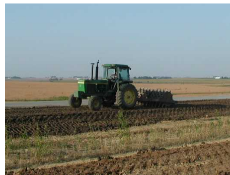
Compaction of earth shoulder material
