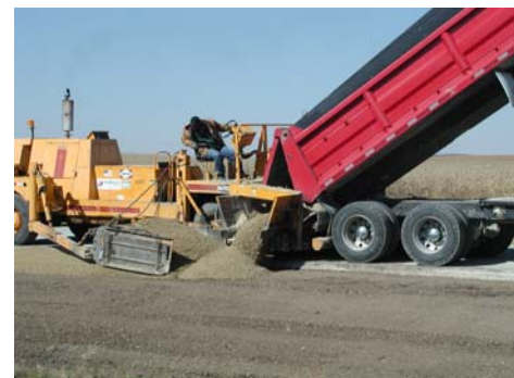
The granular material is placed with a shouldering machine
