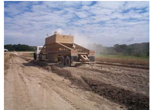
Spreading the fly ash
