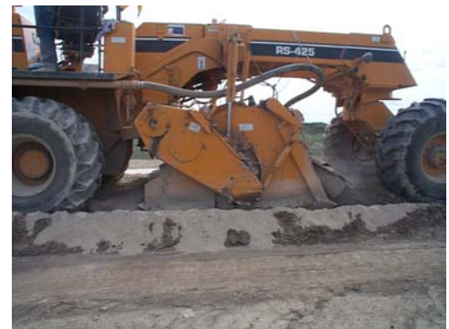
Mixing the fly ash with the soil
