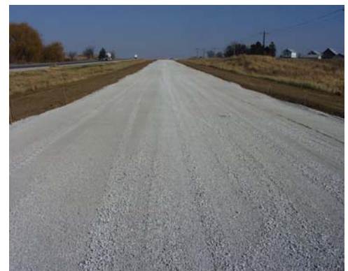
Granular subbase in place
