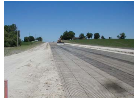
Polymer grid in place prior to spreading of the granular subbase
