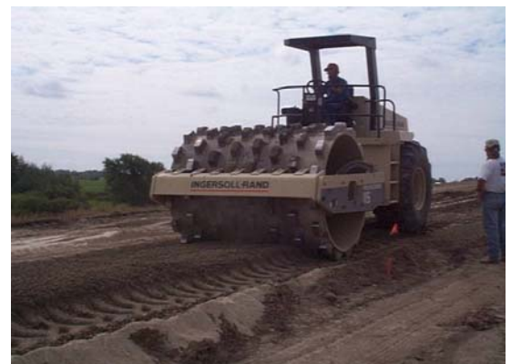
Compacting the fly ash treated material
