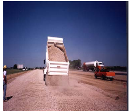
Placing granular subbase
