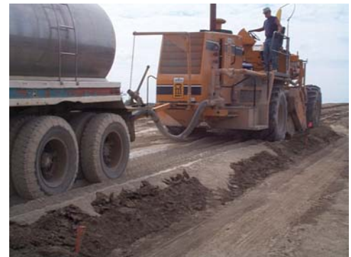
Adding water to the fly ash
