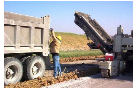
The spreader belt can be dangerous
