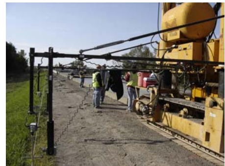
Offset string line reduces potential for tripping
