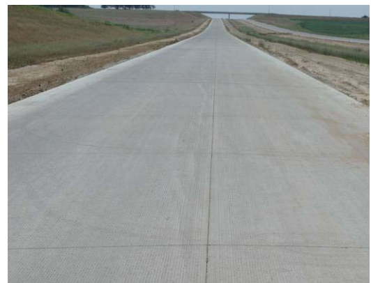
Longitudinal joint on the roadway centerline
