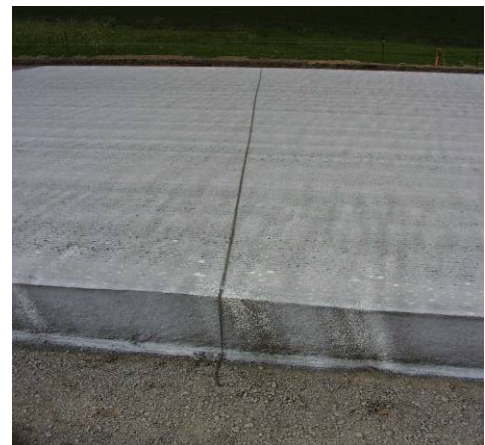
Transverse joint with 6 to 1 skew
