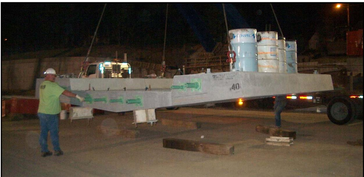
b) Sand-filled barrels were used as ballast during the erection of 40<sup>th</sup> Street Bridge panels
