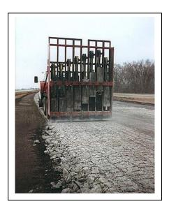
is normally greater. The increased effort is necessary because the original pavement typically contains steel reinforcing bars or wire mesh reinforcement. In order to reduce horizontal slab movements, all slab reinforcement in the PCC pavement must be broken and/or the concrete to steel bond must be destroyed for this technique to be truly effective in eliminating reflective cracking. The Break and Seat technique is considered applicable to jointed reinforced concrete pavements.
