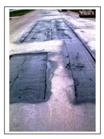
inch but less than the total thickness of the old pavement. The areas are cleaned, tack coated and filled with hot mix in lifts not to exceed three inches. A weighted pneumatic tire or mechanical tamper may be used to compact the mix. The final compacted surface shall be level with to 1/4" above the surrounding surface.
