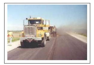
The process is typically used in situations where the existing pavement has surface irregularities, such as minor rutting, oxidation or raveling, but remains structurally sound.
