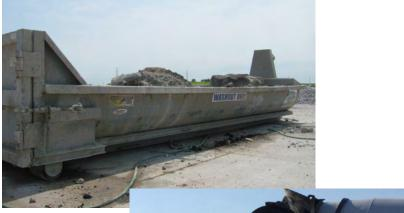
A concrete washout may look like these photos or be as simple as a hole dug to contain the washout as long as it does not adversely affect a water of the state.
