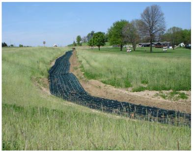
Here TRM was used in a ditch that has potential for high velocity flows.
