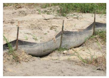
Silt fences at capacity should be noted on the weekly inspection report as a deficiency.
