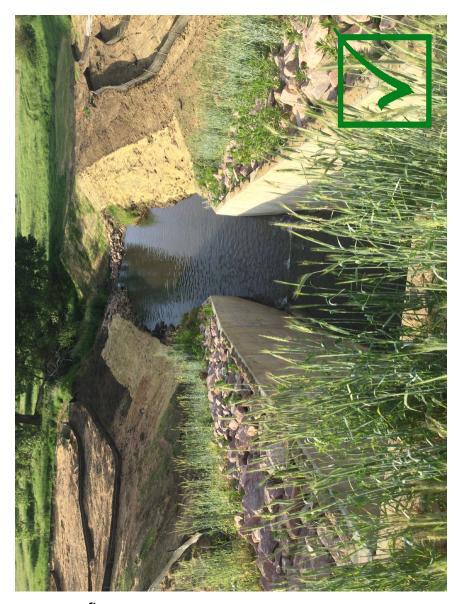
Pipe culvert with multiple controls of rock, slope protection, silt fence and sediment logs.
