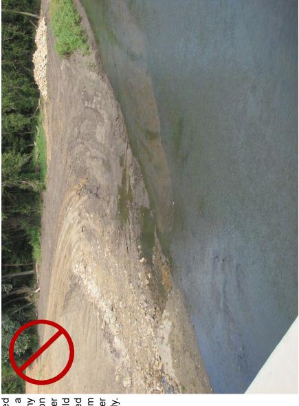
This is a disturbed area alongside a creek without any sediment or erosion controls. Perimeter controls should have been installed to prevent silt from entering the water body. Slope protection was installed on this bridge berm. Silt fence was also installed to control silt from entering the river and to separate the area that was matted from disturbed areas.
