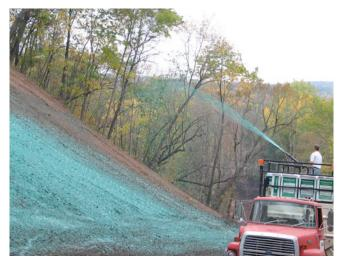
Hydraulic seeding - Typically, inoculant, seed, and fertilizer are to be applied in a single operation. Hydraulic mulch is then applied as a separate operation. Seed conditioner requirements are included in Specifications Section 2601 and Materials IM 469.02.
