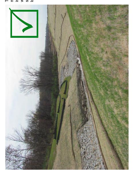
This is an example of a good temporary stream crossing per EW-401. Clean fill was used in the creek, and the crossing was topped with aggregate.
