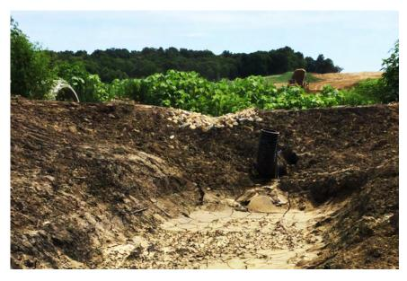
Above, inlet of riser pipe and berm with rock overflow.
