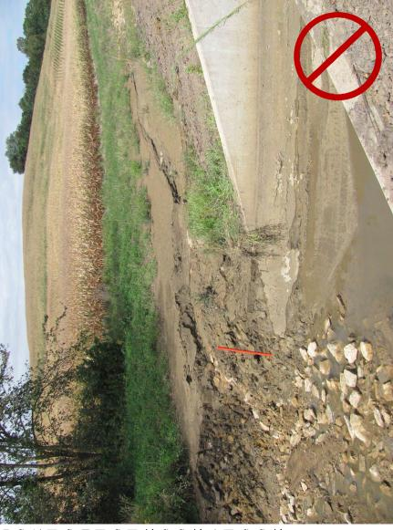
This photo was taken shortly after the outlet end of a box culvert was cleaned out. Based on the silt still remaining in the ditch and the ditt line on the culvert, it's estimated about two feet of silt was removed. The entire site should be reviewed to find what structural controls are needed and areas that should be stabilized. A single silt fence will not prevent recurrence. This site used multiple controls, including silt fence with J-hooks, mat, staged seeding, logs and rock.
