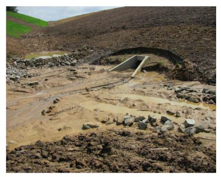
The controls in this area are inadequate. This culvert and basin must be cleaned out, and the slopes need seeding, mulching, and additional silt fence. Form 830245 11-18
