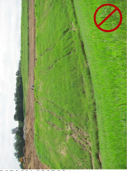
Water drained off the top of the embankment and created rills in the foreslope. This is an example of how an area may appear stabilized but is still susceptible to erosion. These areas should be repaired and if possible, flows should be diverted to a stabilized area. This trench was dug to divert flows down a rock flume and allow vegetation to grow on the slope.
