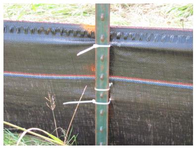
This silt fence was tied with the correct number of ties, but the top tie does not encompass the belt and the bottom tie should be about 4" from the ground.
