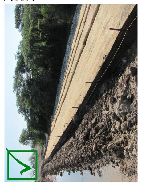
A stream diversion channel was constructed so that the contractor could install a new culvert. This photo shows no controls along the top of the channel (on the left) and spoil piles without silt fence or logs and no stabilization (on the right side of the channel).
