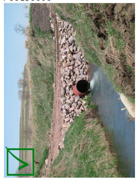
This photo shows a very poor example of a temporary stream crossing on a culvert extension project. Only clean fill per EW-401 should be used in the water.
