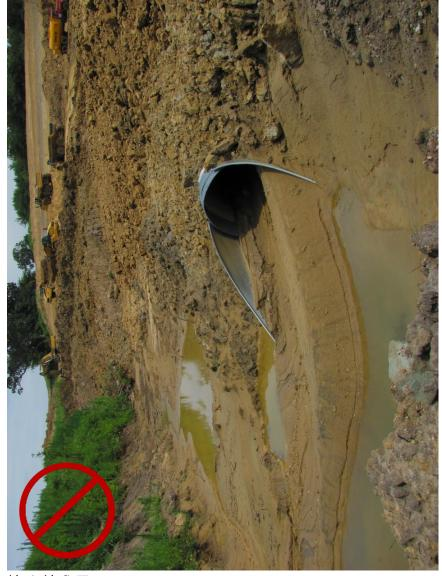
This pipe culvert has no controls around it. A silt basin and silt fence are recommended controls for this area.
