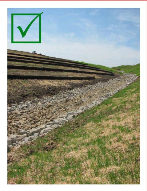
Multiple rows of silt fence installed along the contour of a slope. Due to the ditch grades, a rock ditch was installed to prevent erosion in the ditch. The backslope was also seeded prior to the road embankment being completed. This box culvert has no controls installed. Even if this is immediately after topsoil has been placed, there should be a line of controls installed prior to the waterbody.
