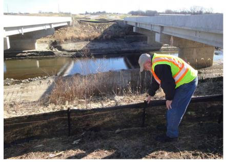
Give the silt fence fabric a good tug to ensure it's properly installed. When properly installed, silt fence fabric should be tight between the posts.
