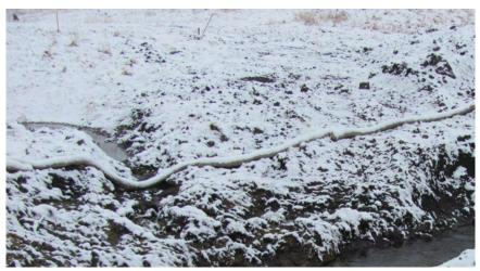
Logs/wattles/socks have the flexibility to be installed in any season. Here a line of logs was installed during the winter to provide protection along a stream.
