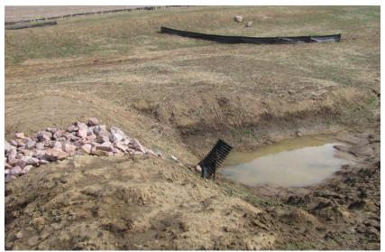
Temporary sediment control basin showing the upstream riser pipe and erosion stone overflow.
