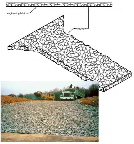
A stabilized construction entrance is designed to minimize tracking of sediment from the site by vehicles and equipment.
