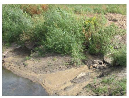
This pipe outlet does not have a splash basin, and erosion is occurring.
