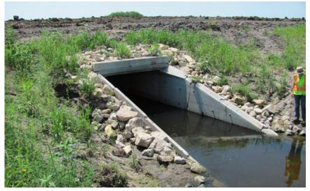
Washouts along culverts and bridges should be repaired before they turn into gullies, such as shown in the photo. The slope should be repaired and seeded.
