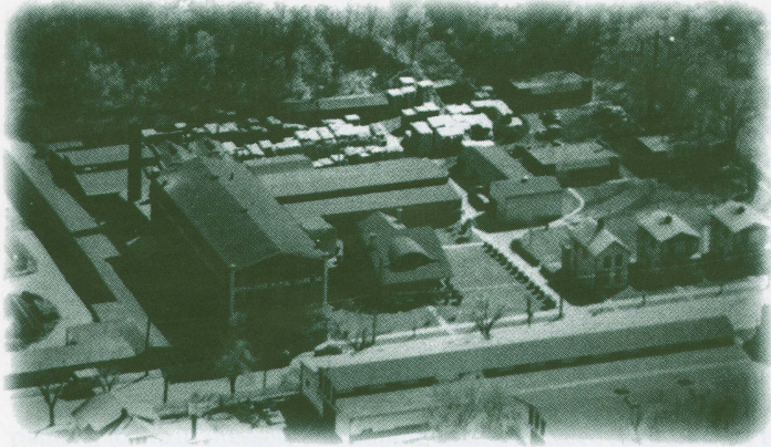
Aerial photograph of the Embalming Burial Case Company in 1940s-mid 1950s. Note the rows of factory workers' houses and the cluster of duplexes along the right side of the photo. (Collection of Murray Turbomachinery Corp., Burlington, Iowa)
