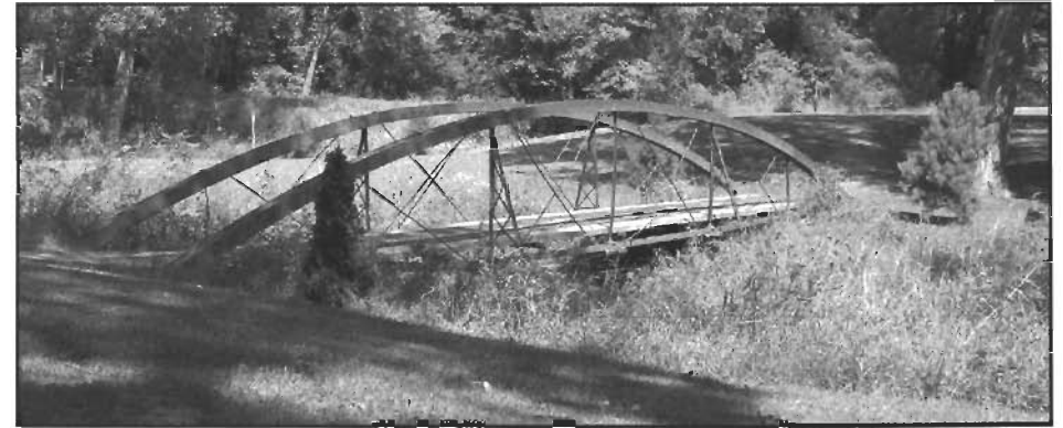
Profile of the the Coon Hunters' Bridge. Photograph by Evan Vulich 2003.
