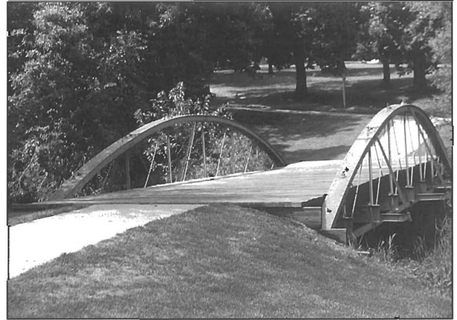
Approach to the Nodaway River Bridge. Photograph by the author 2002.
