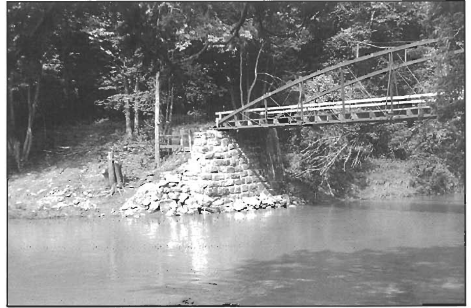
Stone pier repaired at Corbett's Mill Bridge, 2002. Photograph by the author 2002.
