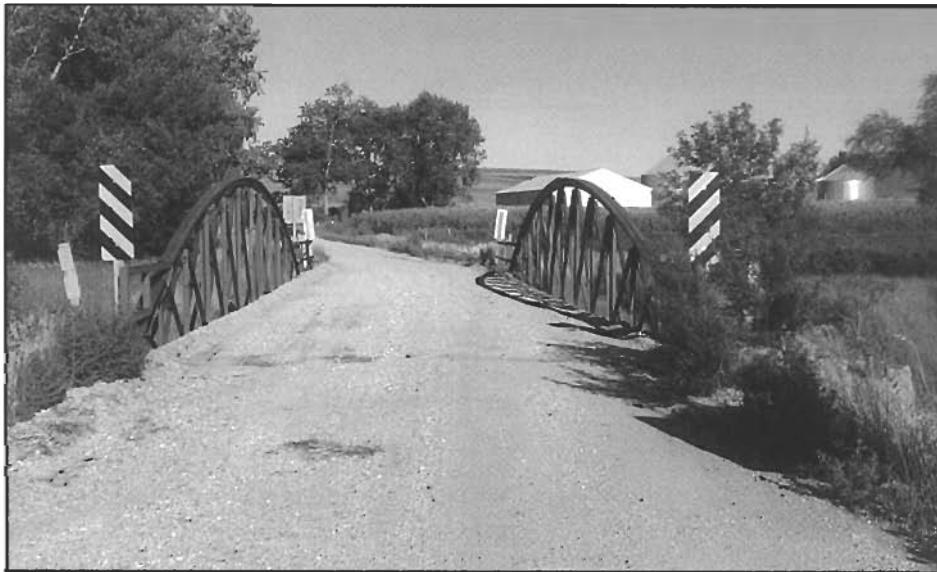
Approach to the Nishnabotna River Bridge, Crawford County, built in 1945. (FHWA#: 126410)
