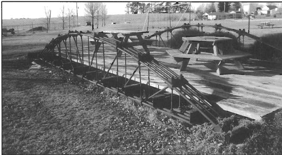
Profile of the Eureka Bridge, Winneshiek County, built in 1871. The bridge is located in the City Park of Castalia. Photograph by the author 2002. (FHWA# none)
