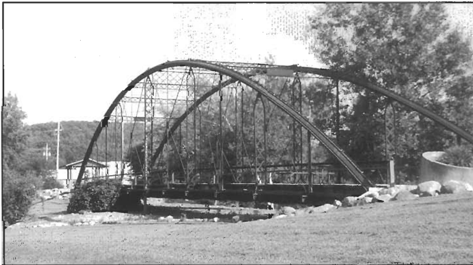
Profile of the Freeport Bridge, Winneshiek County, built in 1878. The bridge is located in Trout Run Park, Decorah. Photograph by the author 2002. (FHWA#: none)
