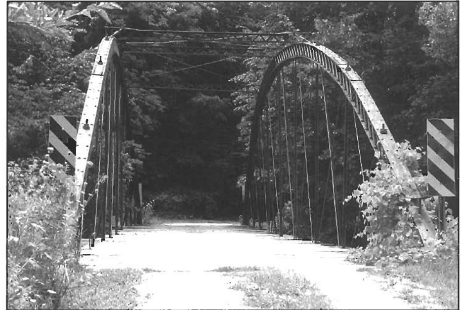
Approach to the Washington Mill Bridge, Dubuque County, built in 1878.
