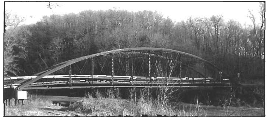
Profile of the Gilliece Bridge. Photograph by the author 2002.
