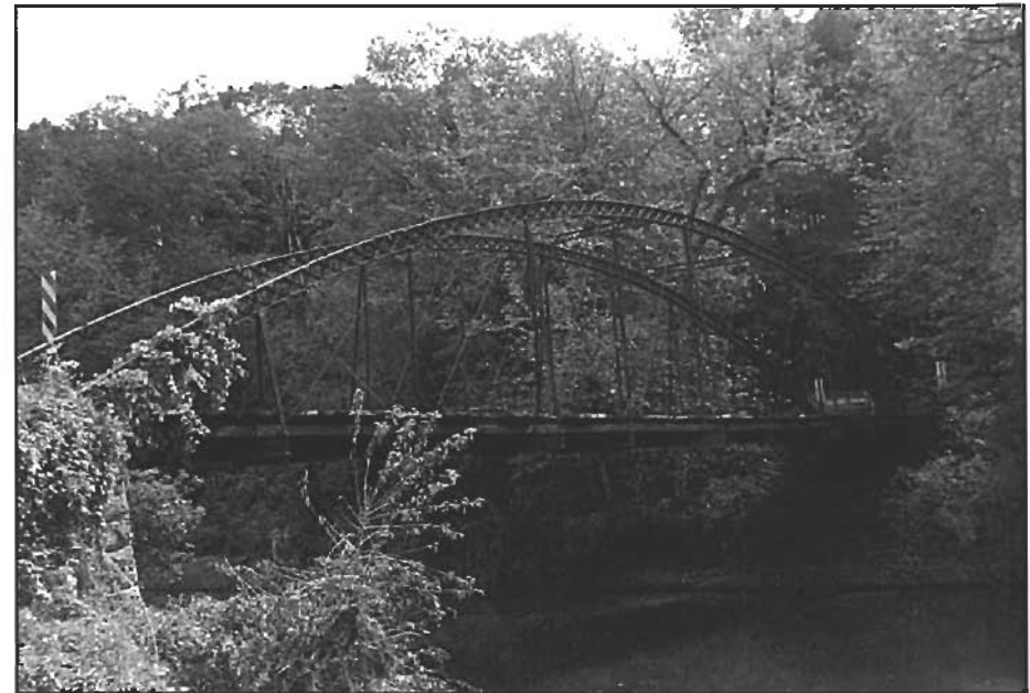
Profile of the Washington Mill Bridge. Photograph by the author 2002.
