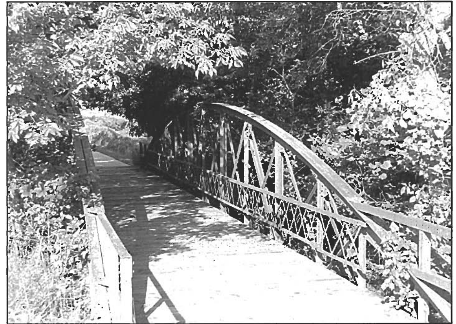
Approach to the Yellow Smoke Park Pedestrian Bridge, Crawford County, built in 1945. Photograph by the author 2002. (FHWA#: none)
