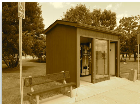
Early vending machine building at the northbound rest area in Woodbury County on Interstate 29.
