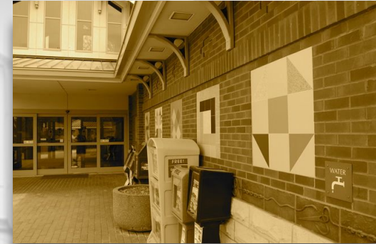
Tiled quilt murals were integrated into the exterior restroom building cladding, as well as the picnic table canopies, and the flooring in the entry vestibule. Decorative brackets were also utilized under the eaves of the restroom building to further create a depot-inspired environment.
