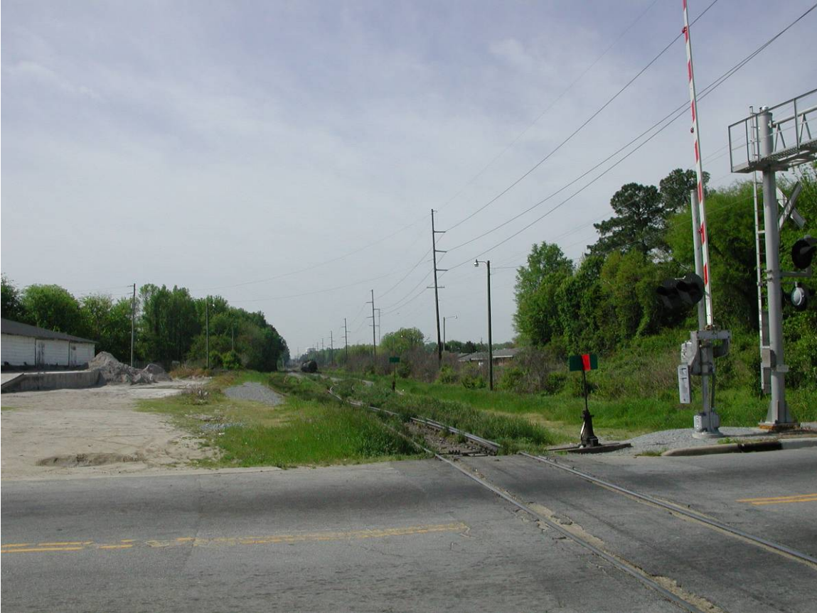
Figure 2. – CSX rail yard and Howell Street
