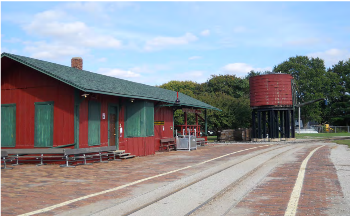
Figure 2.5: Midwest Central Railroad Station Facility
