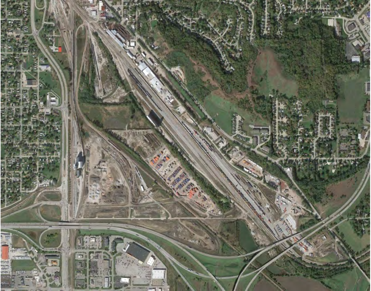
Figure A.11: Council Bluffs Railport
