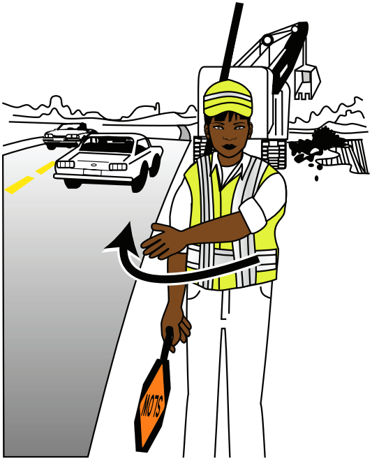
Figure 8 Releasing traffic in a single-flagger operation
